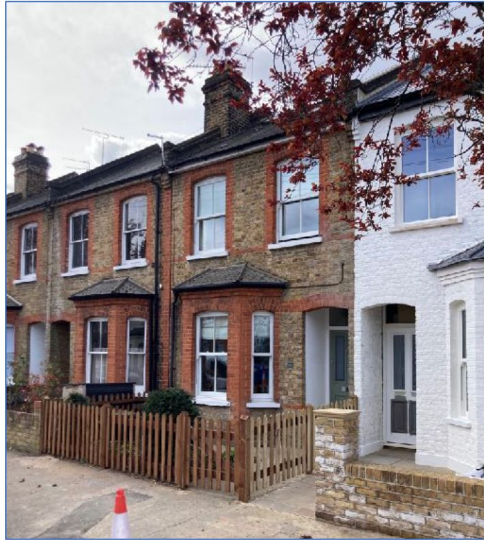
Existing street view of N°41 Arlington Road.
