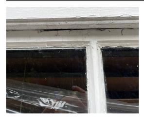
**Front Elevation**Draught through top sash due to defected top rail
