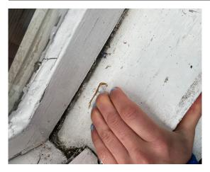
**Front Elevation**Rot to sash window sill, signs of mould
