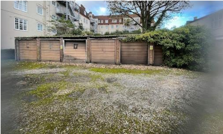
Figure 4.4 Garages and Apartment building
