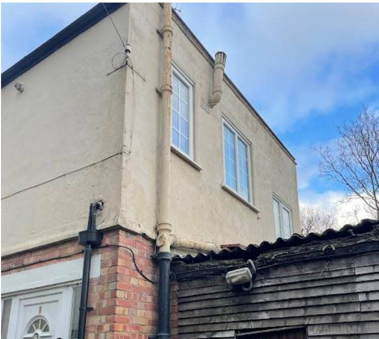
Figure 4.8 Potential ingress points into the apartment building
