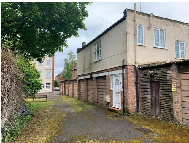
Figure 4.3 Garages and Apartment building
