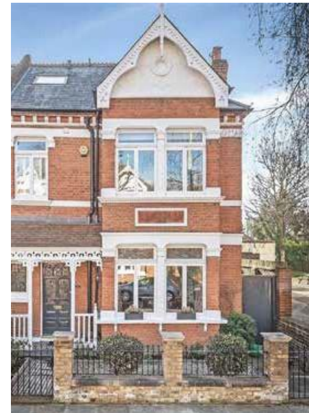
19 Lebanon Park shares a party wall with the garage site.
