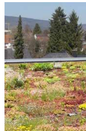
Extensive green roof
