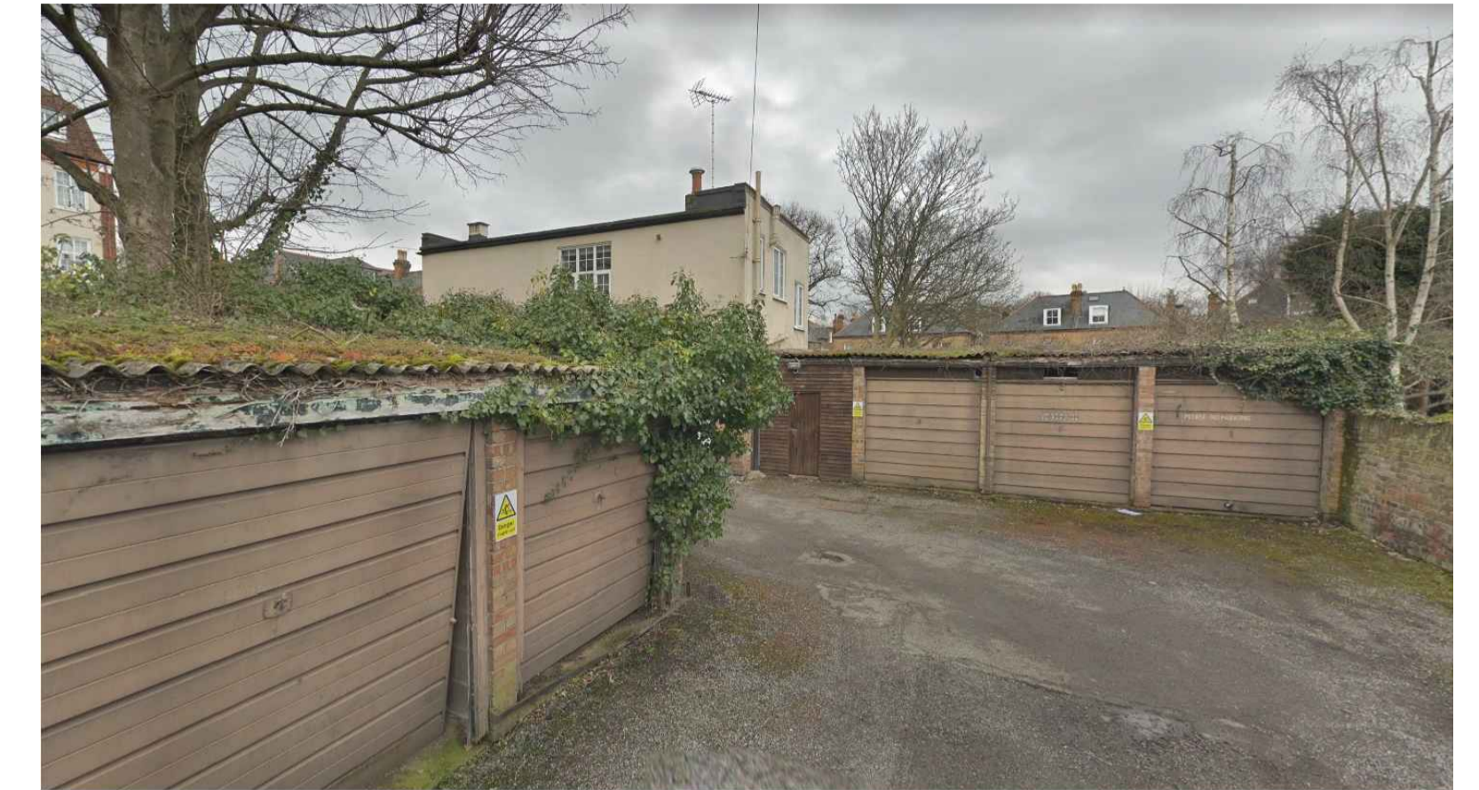
View of Garages & First floor flat from Sion Road access
