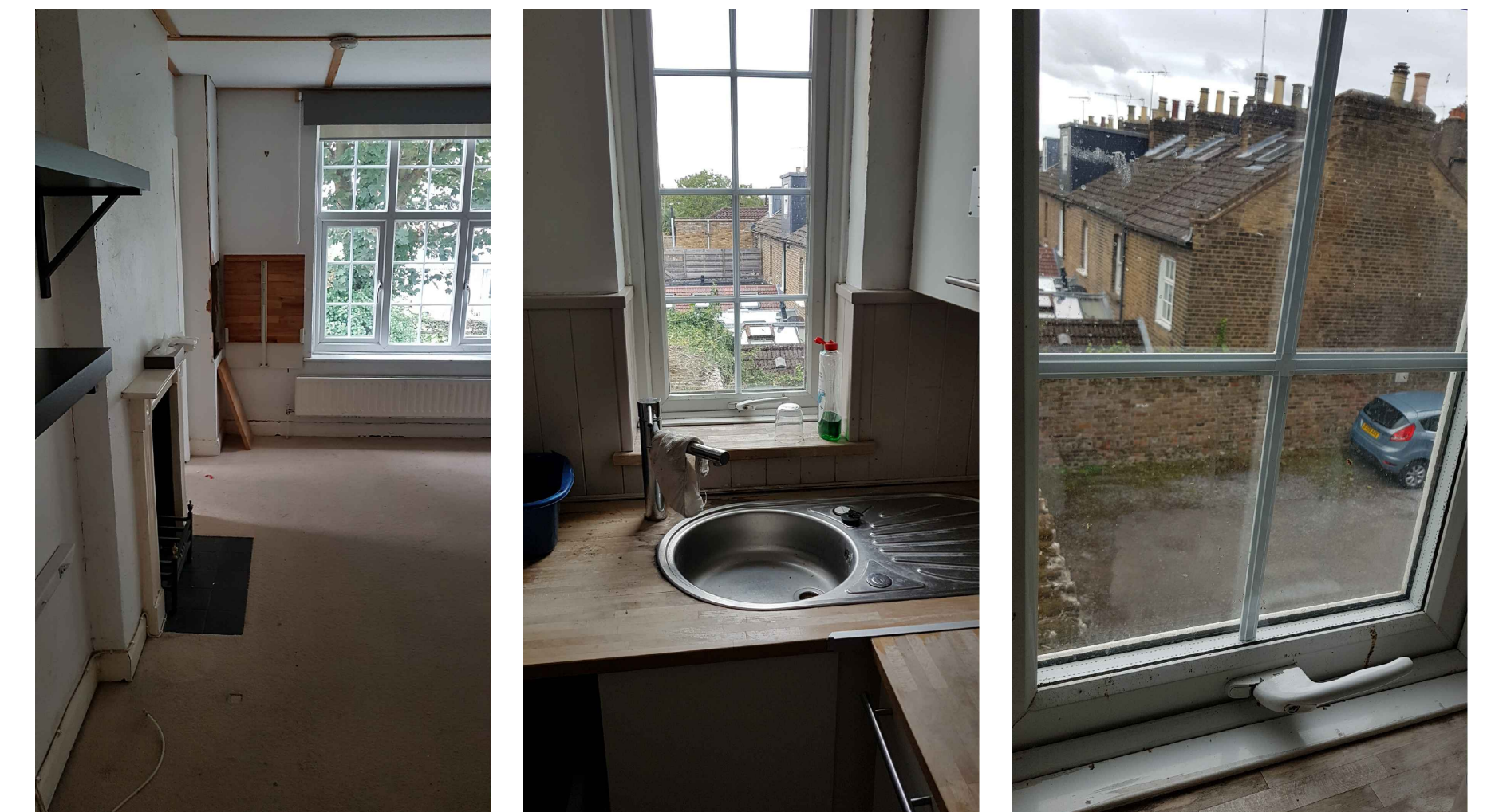
Existing first floor flat & view from side windows
