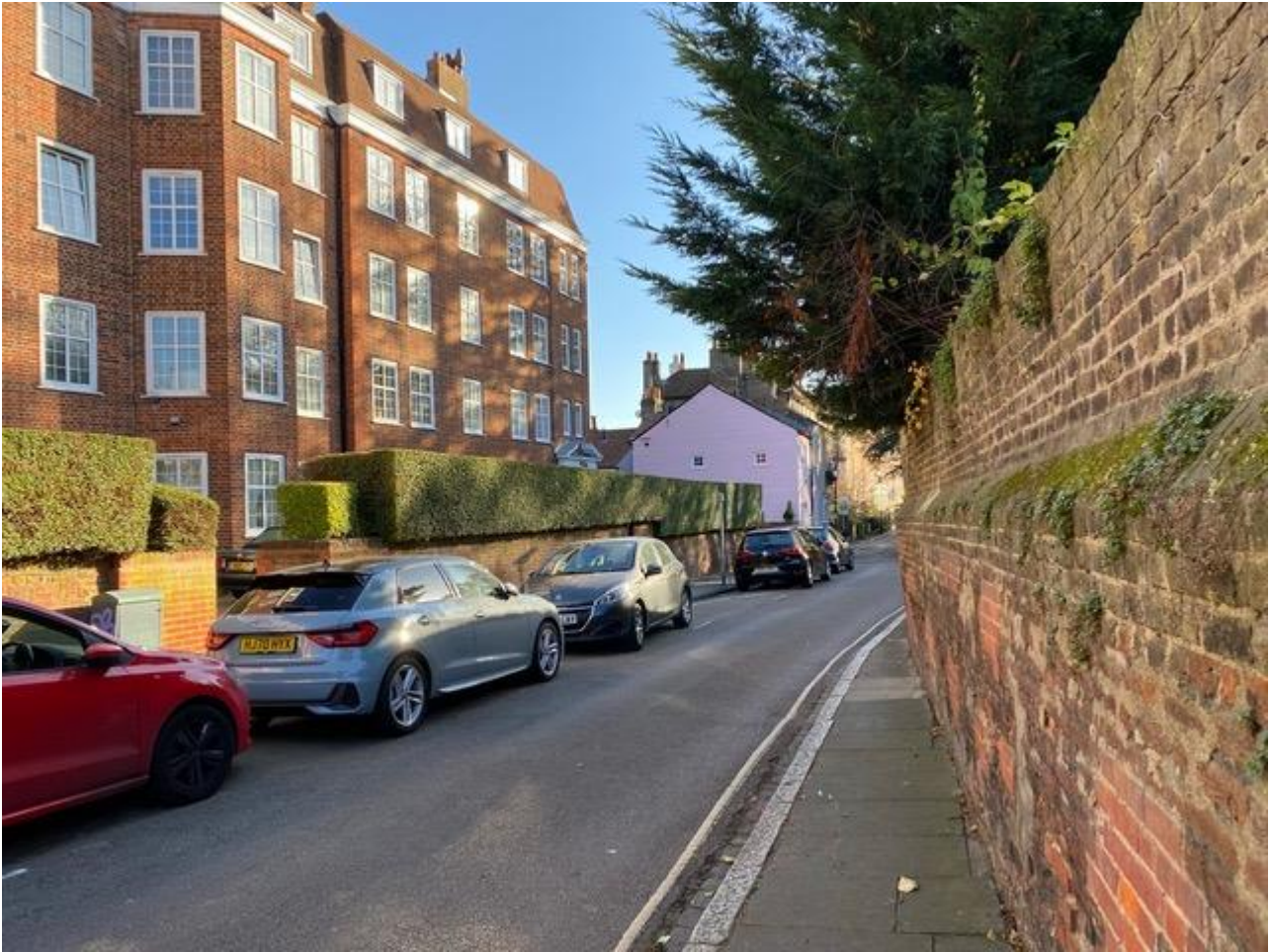
Figure 6 - Looking south-east in Sion Road with Sion Court to the left and the gable wall of 14 Sion Road (locally listed) beyond.
