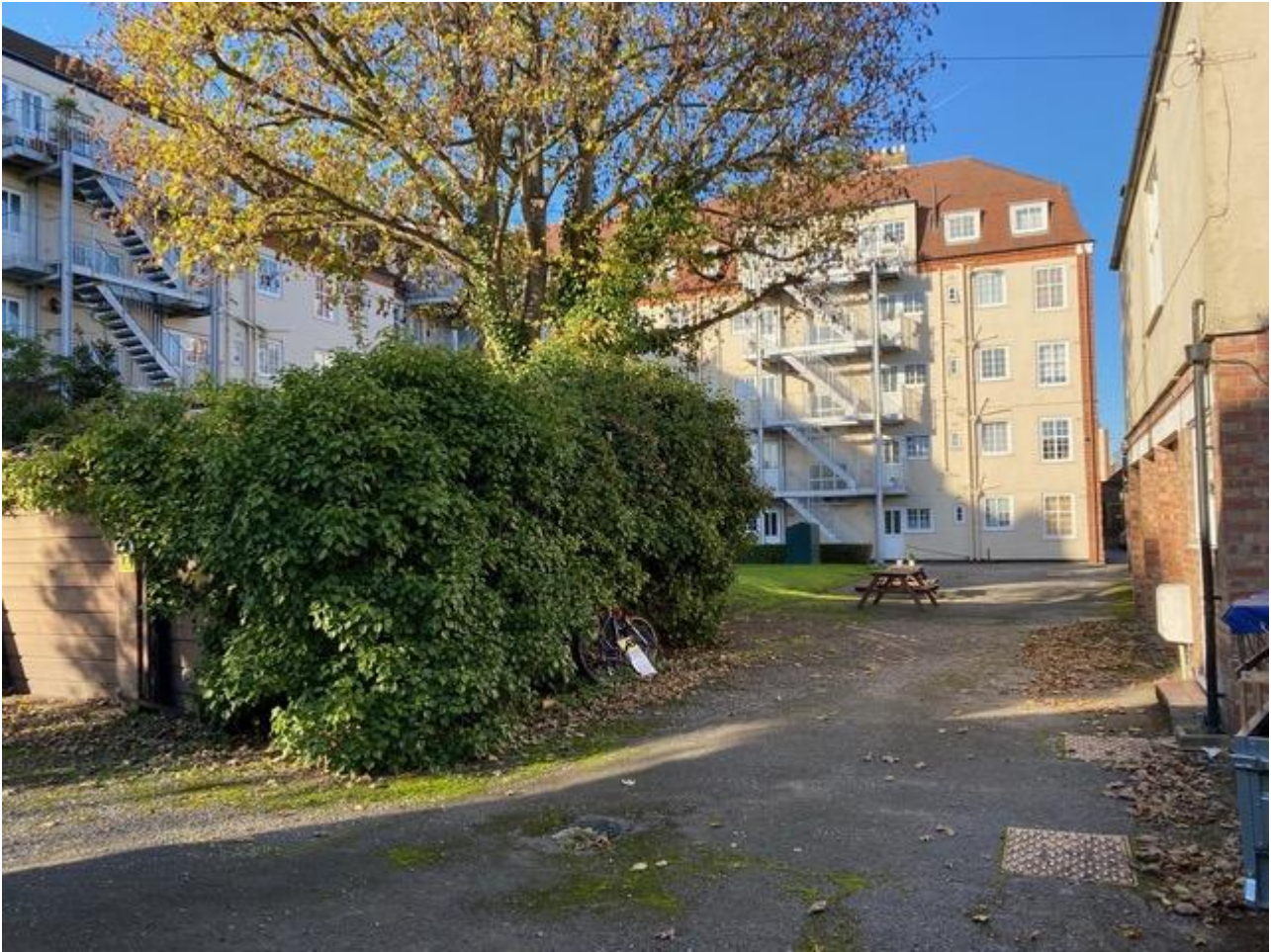
Figure 13 - The back of Sion Court, looking towards Lebanon Park, with the two groups of garages in the foreground and to the right.
