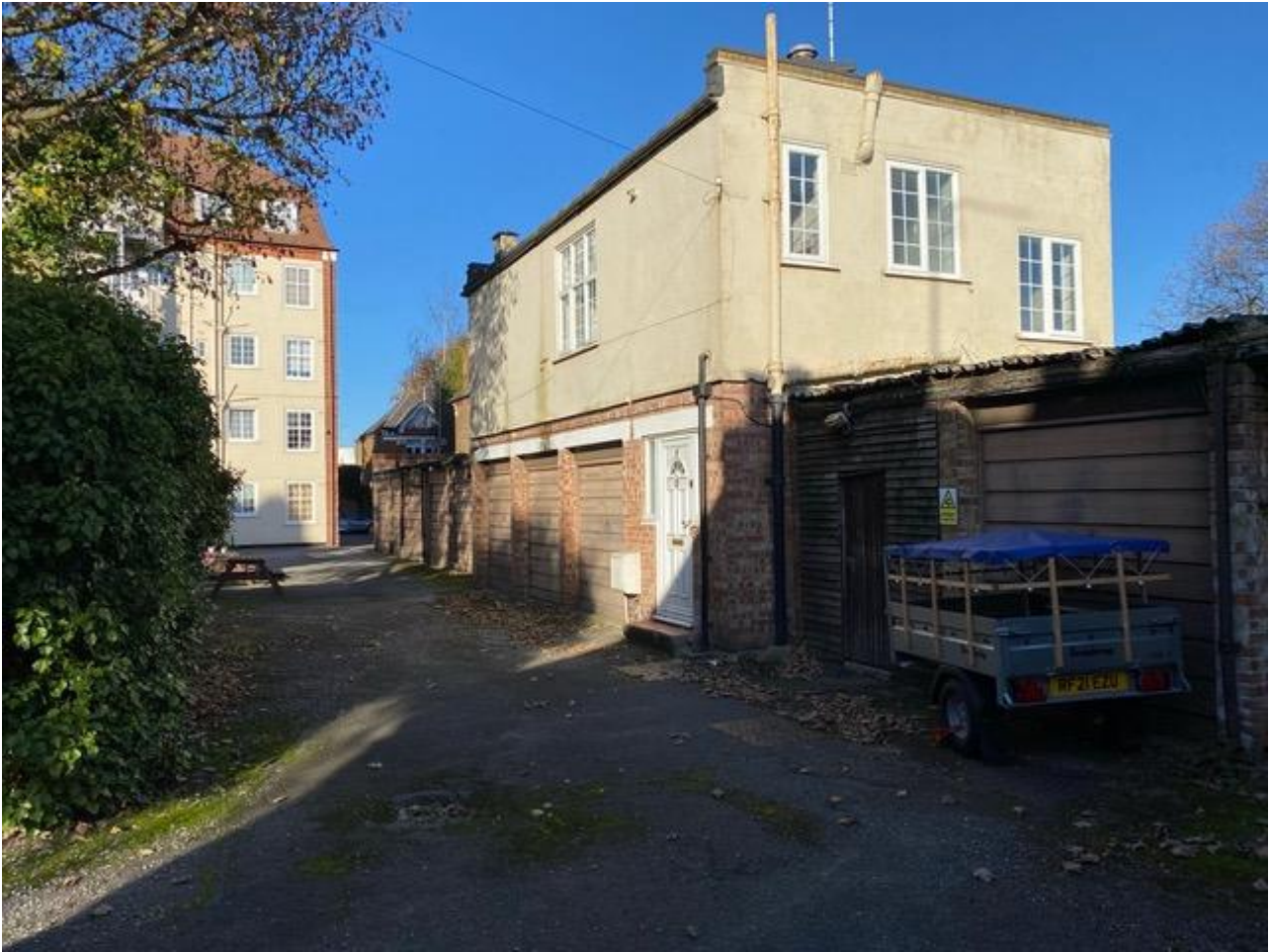
Figure 11 - The first floor residential accommodation over some of the garages. This, and the garages to the right, appears on the O.S. map of 1936.
