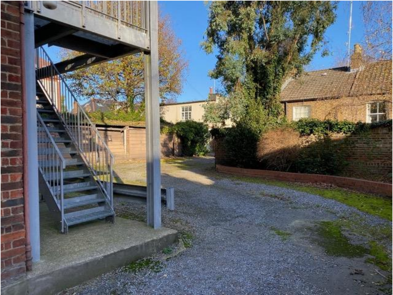
Figure 9 - Looking into the application site from the Sion Road entrance. To the right are the locally listed buildings known as 9 and 11 Ferry Road. The garages and flat roofed first floor accommodation can be seen in the centre-left, beyond the metal staircase.
