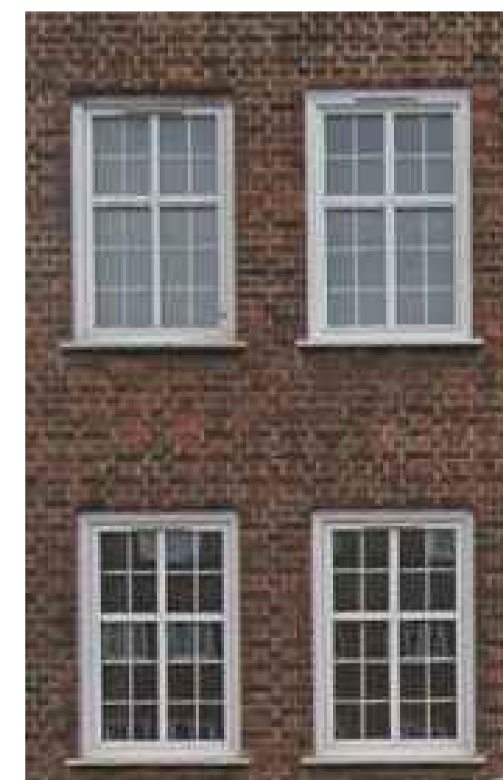
Vertical windows in Sion Court
