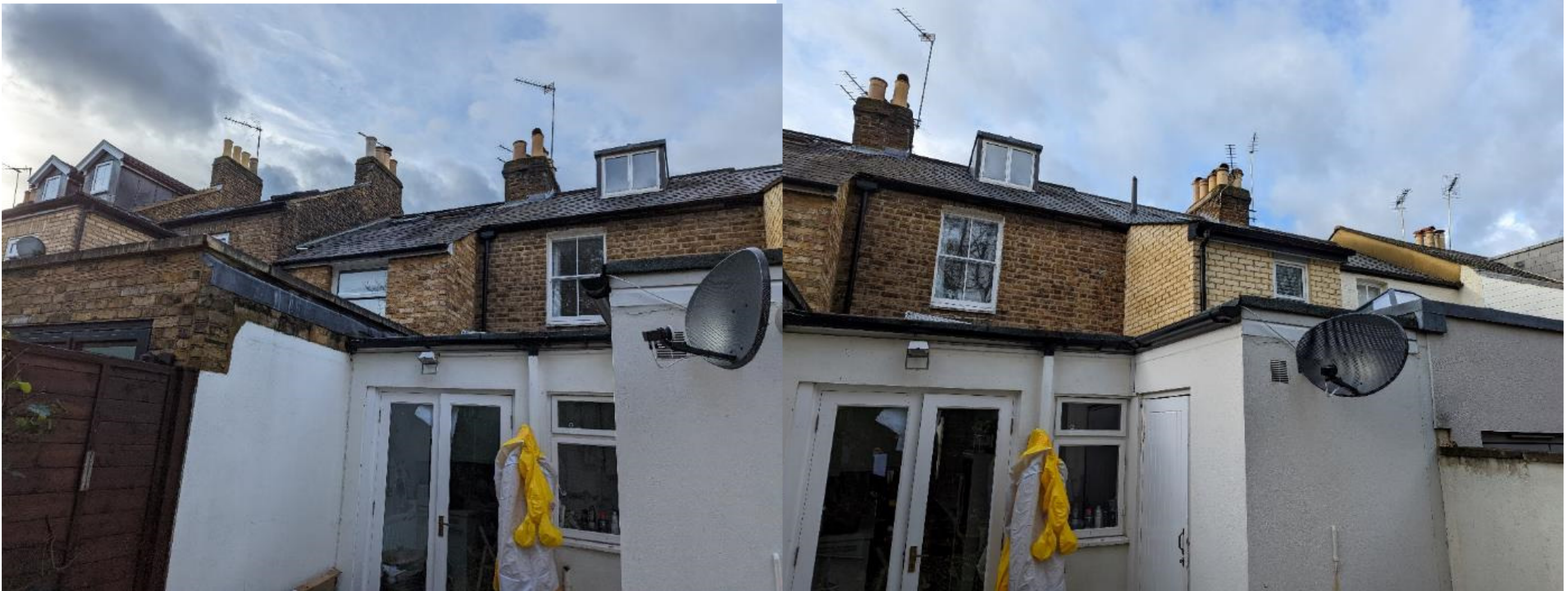
Rear View to No.s 24 & 26
