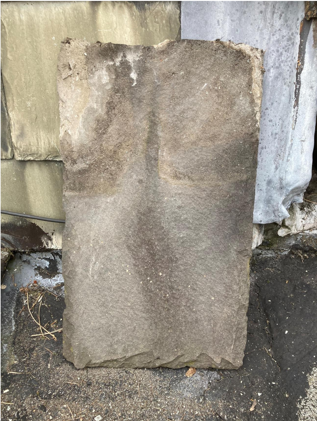
Figure 2: Like-for-Like Slate Replacement
