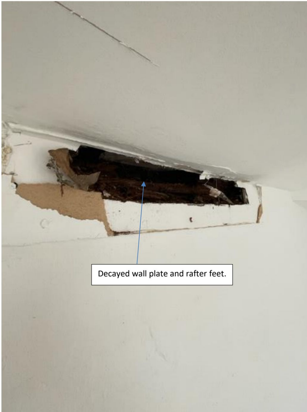
Photo 3 Close-up of decayed timbers
