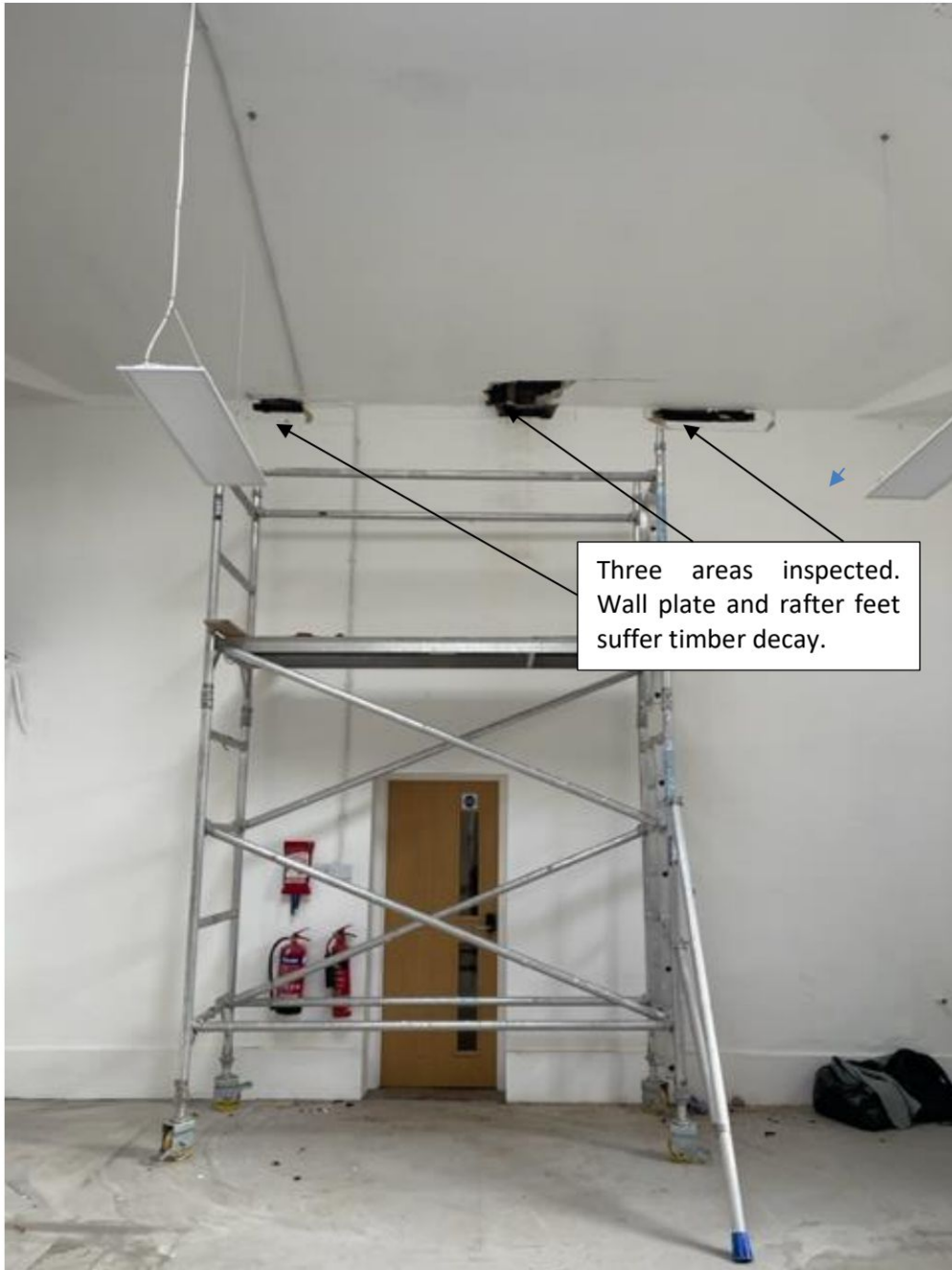
Photo 1 Inspection hole locations
