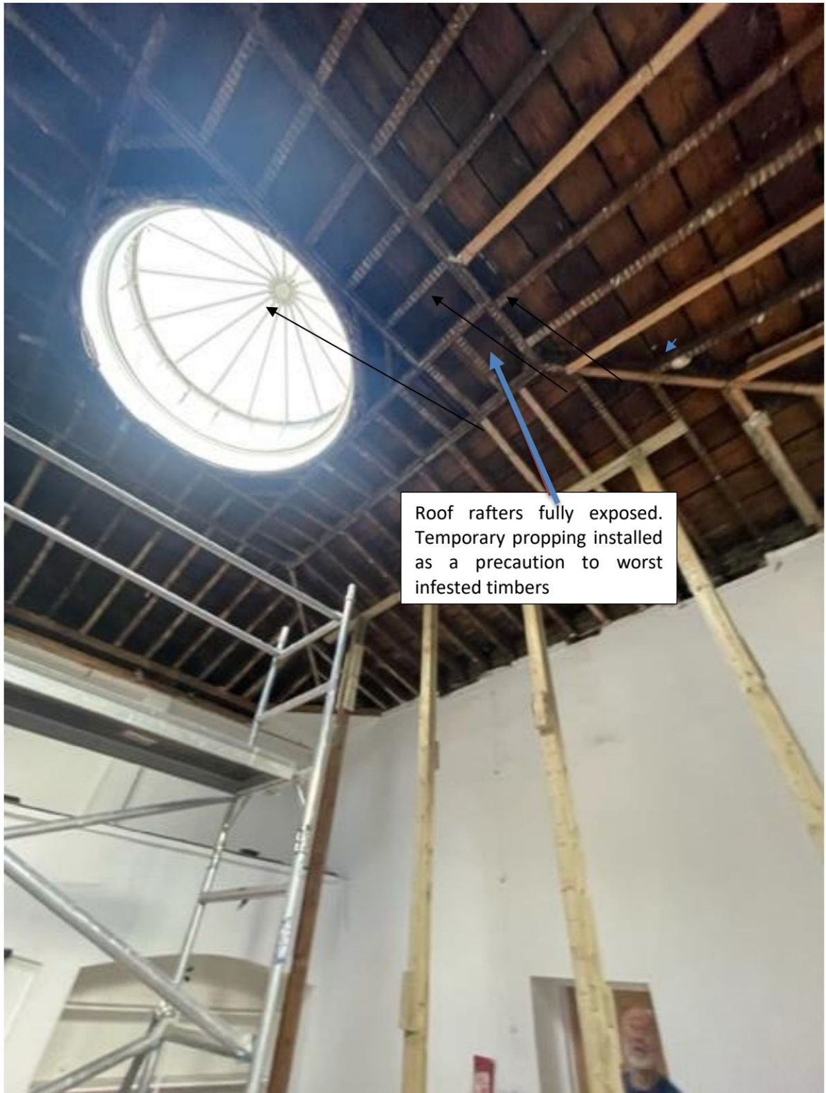
Photo 2/1 Main roof rafters
