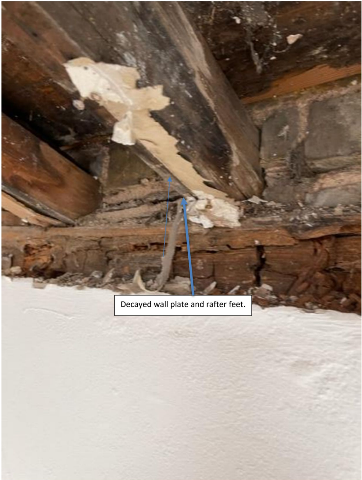
Photo 3 Close-up of decayed timbers
