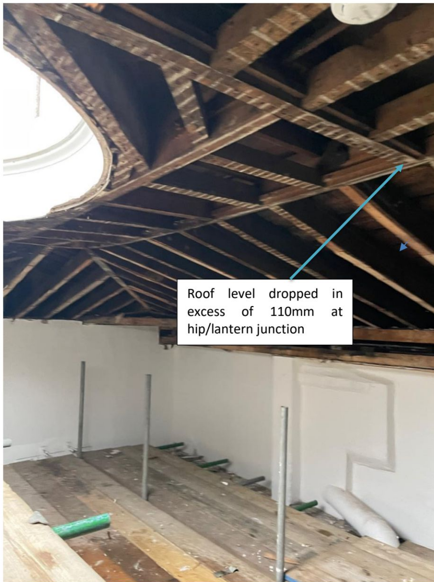
Photo 3/1 Main roof rafters
