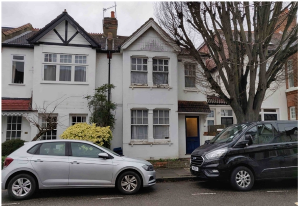
Figure 2 - View of property from road showing sufficient access for fire appliances
