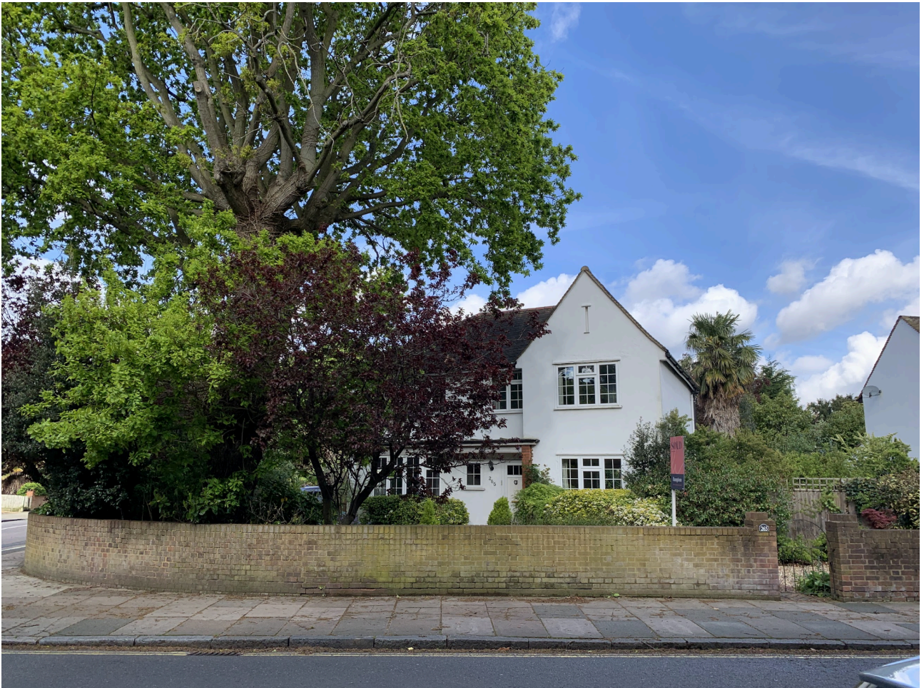
Figure 1: Photograph looking North West at the building frontage showing the existing low brick boundary wall and mature oak tree.
