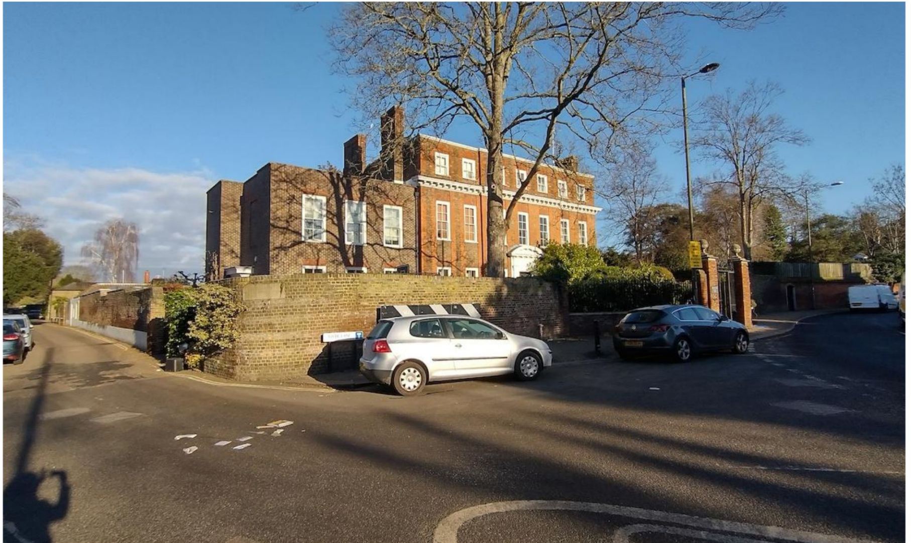
The House 145a, Petersham Road, Richmond, Surrey TW10 7AG Heritage and Design and Access Statement HOU-P-05(B)
