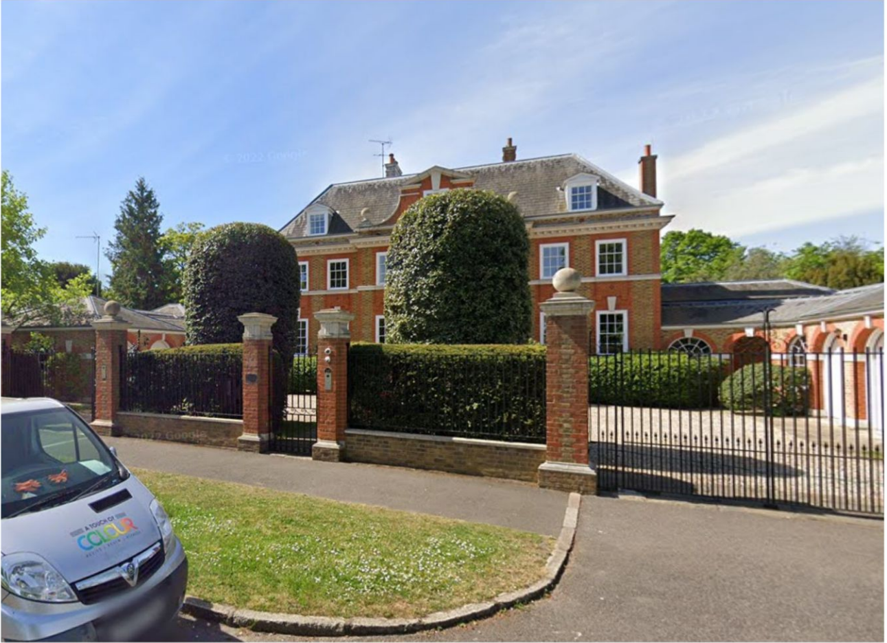
Slate Roof and Small Dormers
