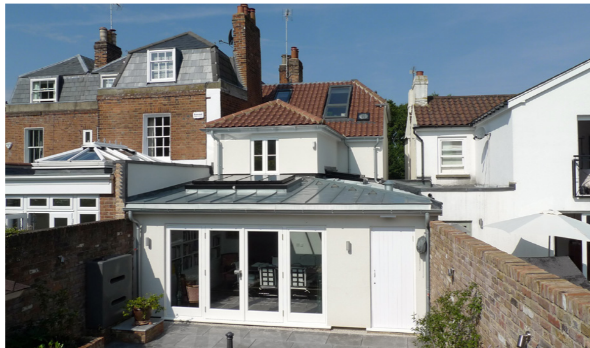
Fig 16. Thames Ditton House - Phillips Tracey Architects: A zinc roof extension to a Grade II listed cottage.
