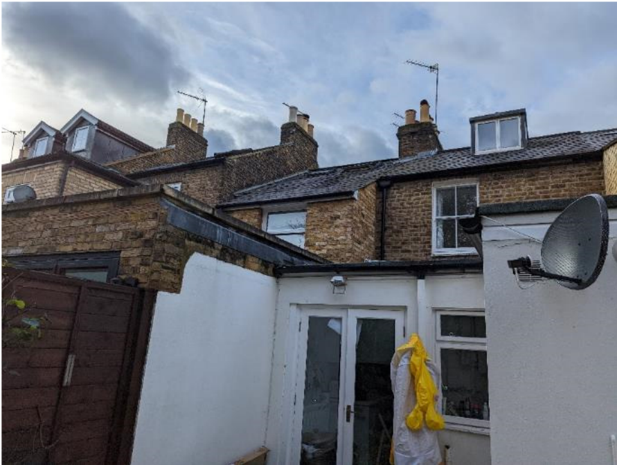
Rear Extensions of house No. 24
