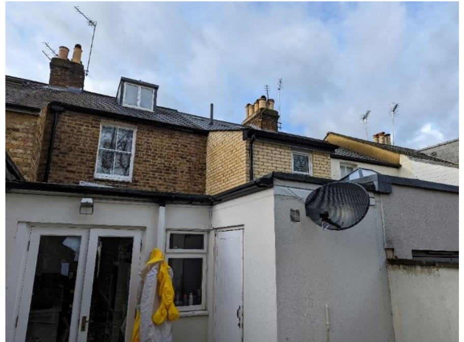
Rear Extensions of house No. 20
