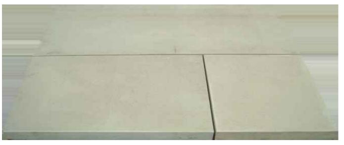
**NEW PAVING TO PEDESTRIAN PATHWAYS:** DIAMOND SAWN MANOR YORKSTONE PAVING BY BINGLEY STONE 50mm THICK SMOOTH FINISH SLABS - SLABS TO BE CLOSE JOINTED
