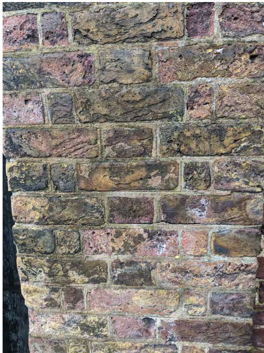
DETAIL OF EXISTING BRICKS ON DOUGHTY HOUSE GATE PIERS
