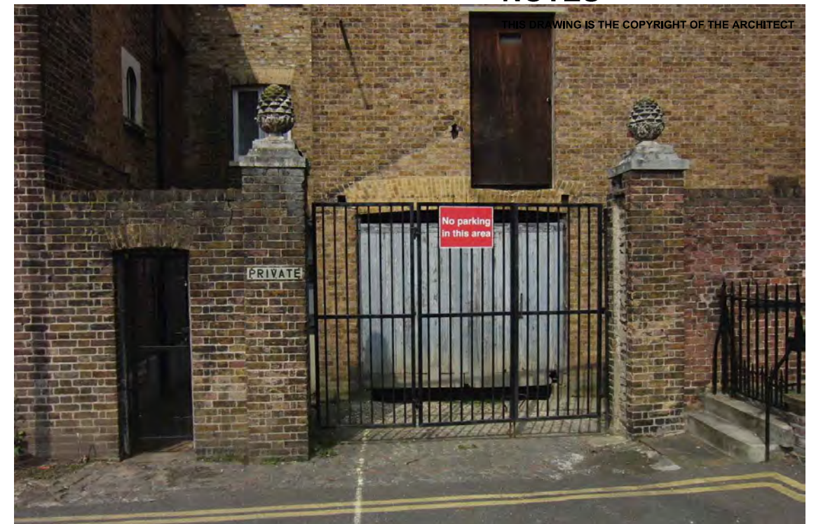
GATE PIERS AND DOUGHTY COTTAGE WALL IN CONTEXT
