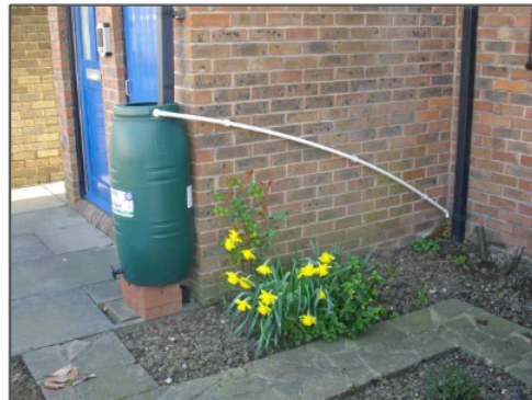
Figure 4-6 Example of a 100L water butt retrofitted to existing development
