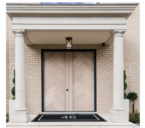
REFERENCE IMAGE, ENTRANCE DOORS
