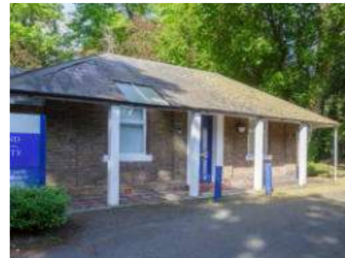
Oak Tree Cottage (locally & curtilage listed)
