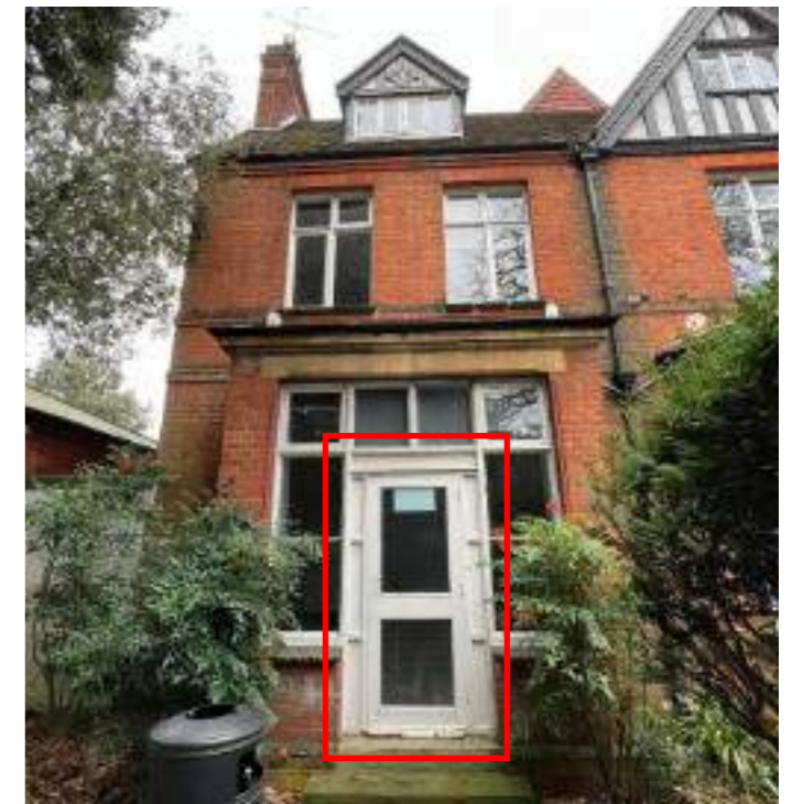
Photograph of door to be replaced
