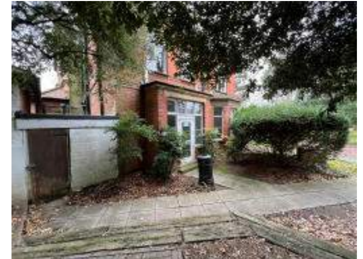
Landscaping required to path to provide level access to the rear entrance
