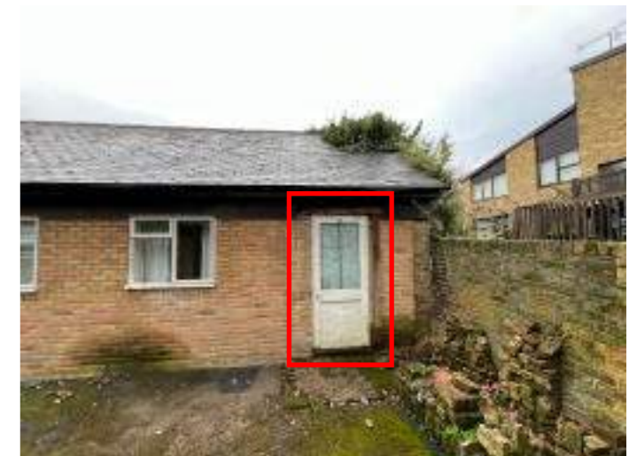
Photograph of existing external door to be altered
