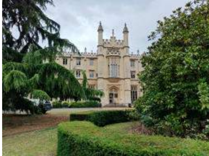
Main Building (Grade II listed)
