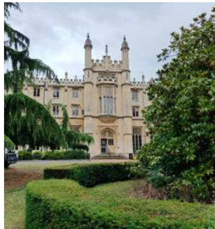
Photograph of main entrance showing stepped approach
