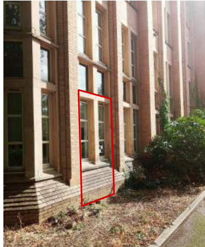
Sir Cyril Taylor Library - existing window opening to be amended to form external door
