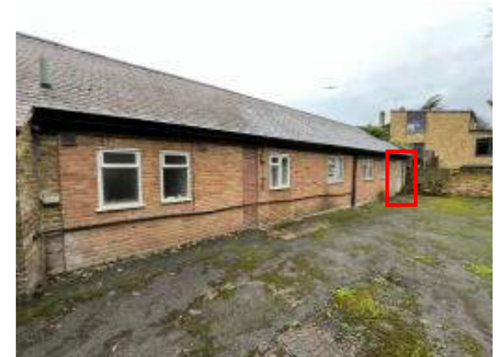
Photograph showing location of existing external door to be altered
