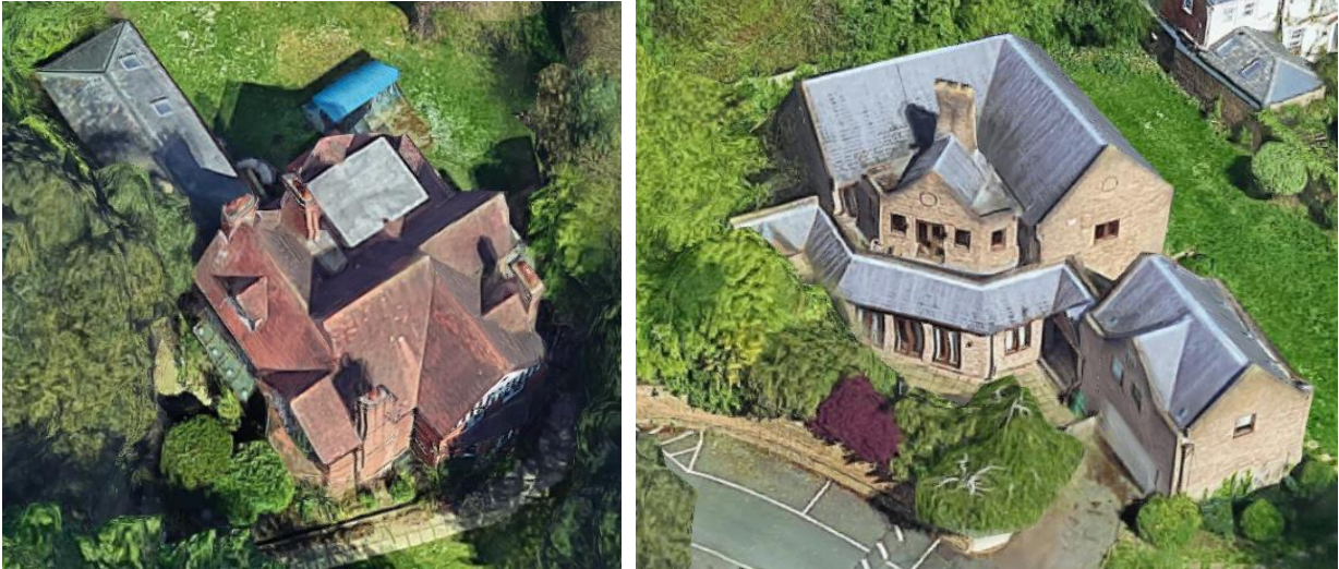
Figure 36 (left): Aerial view of the Red House (Google, 2023).
