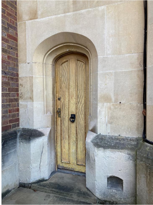
Figure 13: Side entrance door to south-east elevation.
