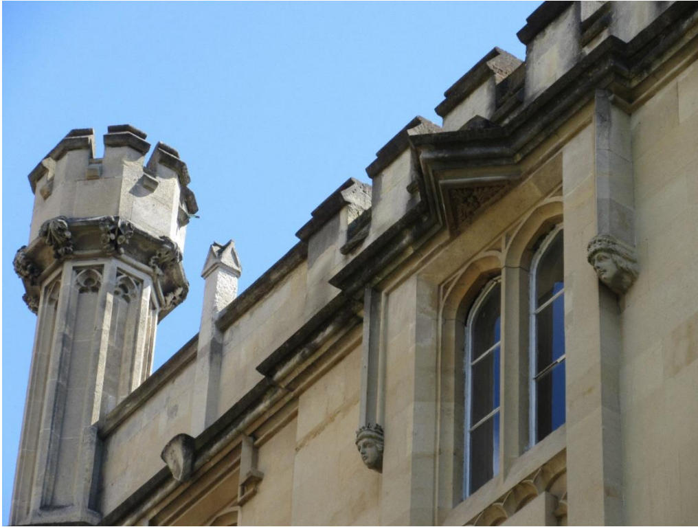
Figure 15: Details of the north-west elevation of the principal building.
