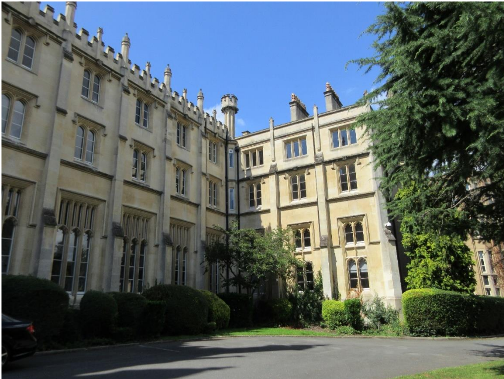
Figure 12: Front (north-east) elevation of central part, and south-east elevation of north wing, of the principal building.
