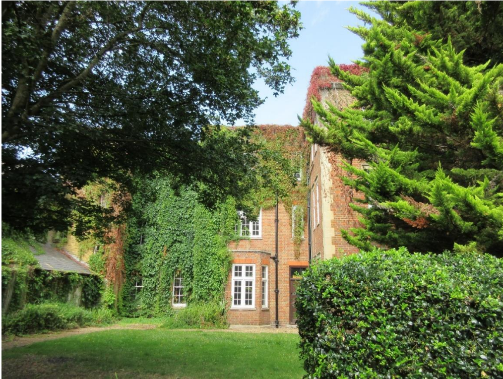
Figure 9: Side (south-east) elevation of George House.
