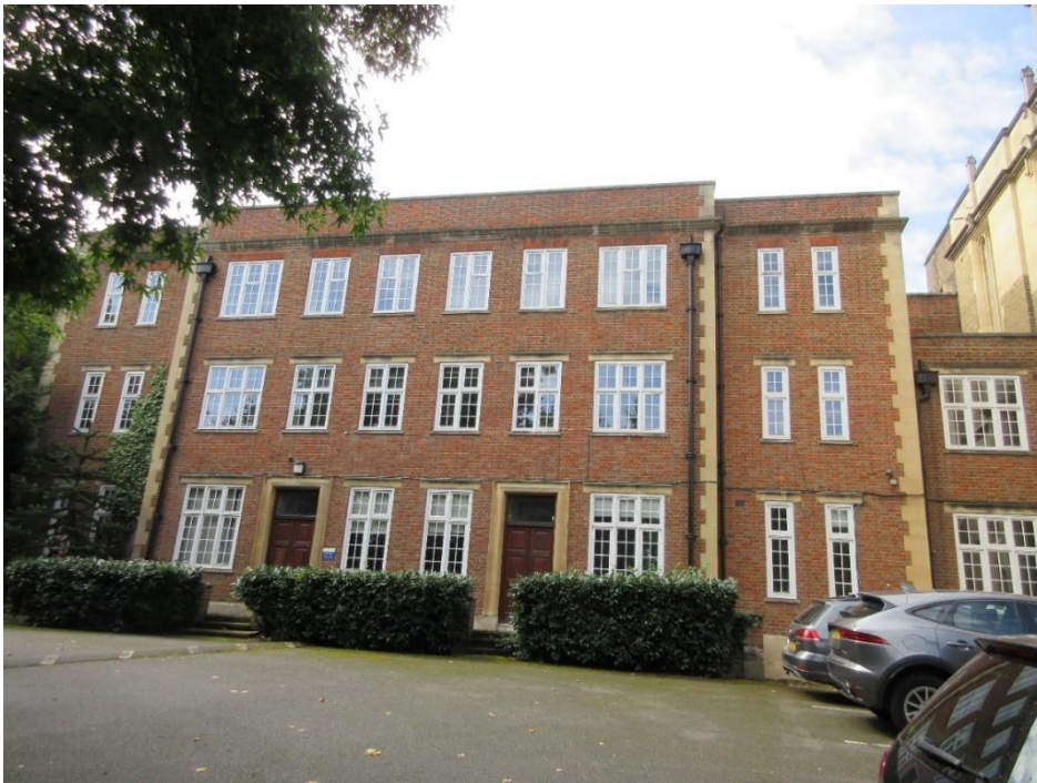
Figure 7 (left): Front (north-east) elevation of George House.
