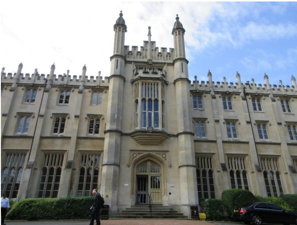
Figure 10: Front (north-east) elevation of the principal building.
