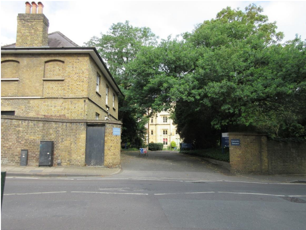
Figure 13: Westward view towards southern entrance to subject site. Lower Cottage (locally listed and curtilage listed) is on the left, and the principal Richmond College building (Grade II) is in the distance.
