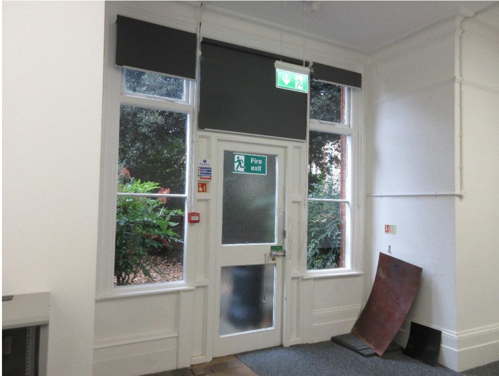
Figure 78: Interior of secondary entrance, located within the south-west elevation.
