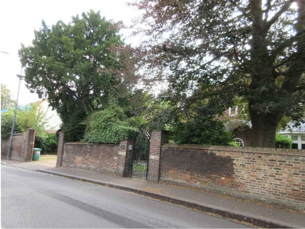
Figure 12: Front boundary treatment of Ancaster Cottage (unlisted) and Ancaster Lodge (locally listed).
