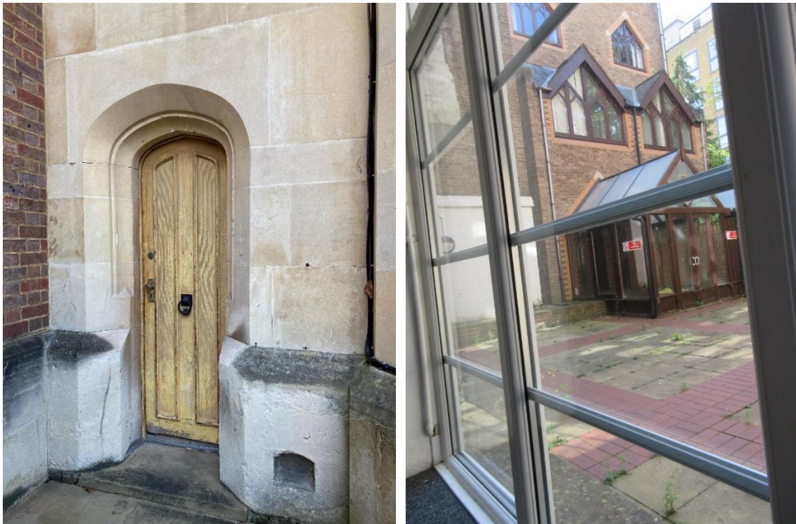
Figure 67 (left): Side entrance door to south-east elevation. (Also Figure 13, Appendix 3.)
