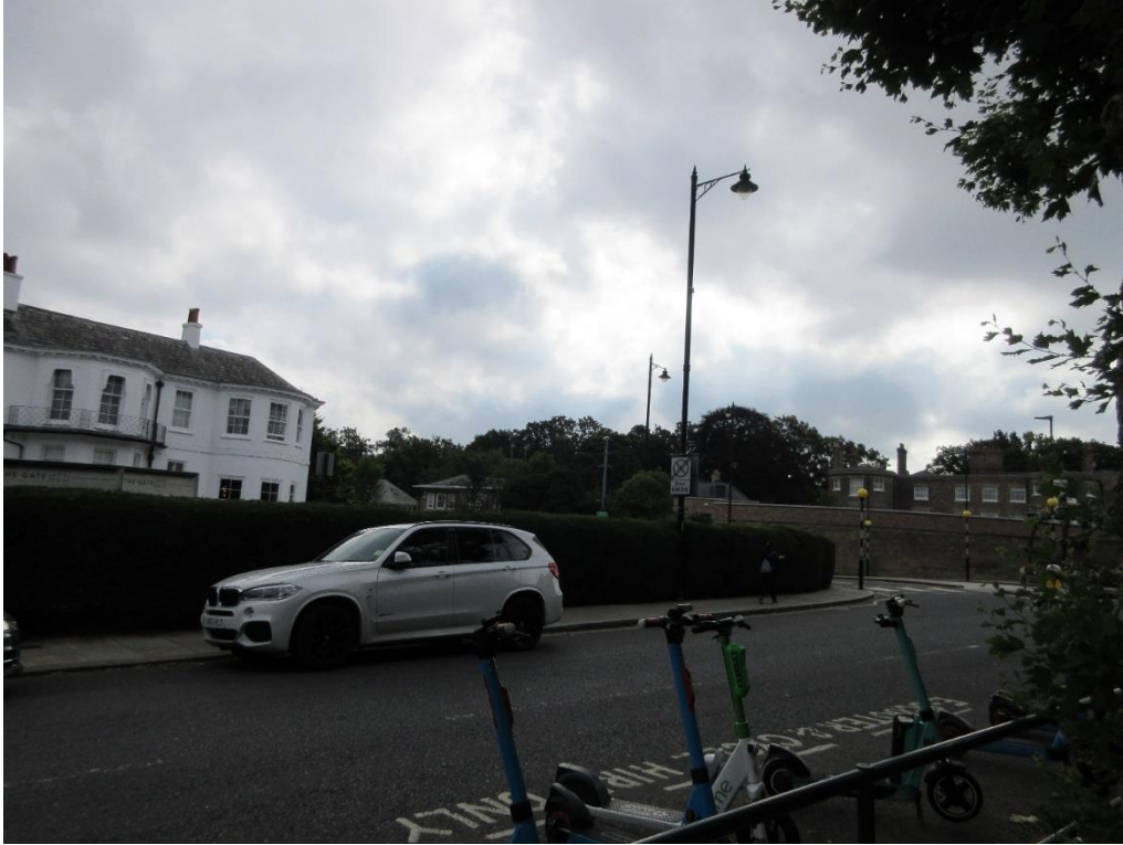
Figure 6: Westward view towards the junction between Richmond Hill and Queen's Road. Richmond Gate Hotel (Grade II) is on the left. On the right are glimpses of the Cattle Fountain outside the Star and Garter Home (Grade II), a wall behind which the single-storey Peregrine Court (unlisted) is located, and Ancaster House and Star and Garter Nurses' Home (Grade II).
