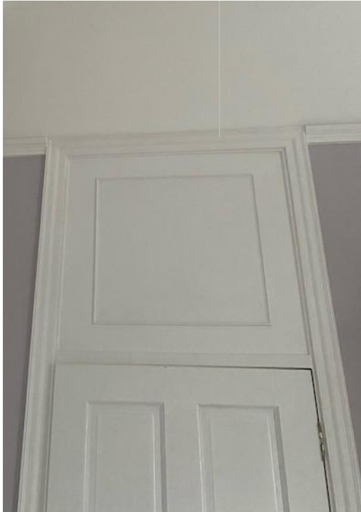
a.glass has been painted to look like timber panels with plant on moulding
