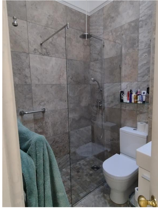
b. existing shower room
