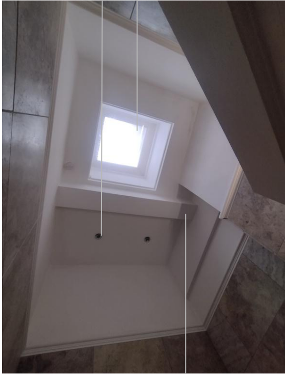
a. existing shower room ceiling
