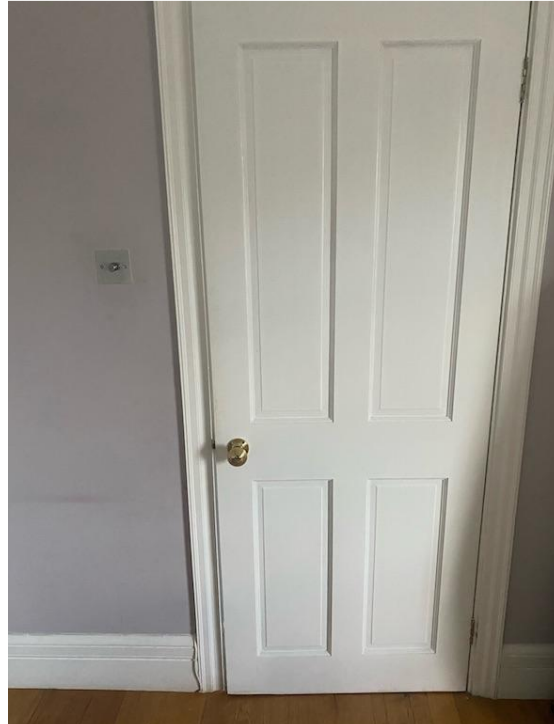
b.existing four panel doors
