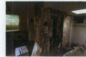
Kitchen area - Minor alterations to internal walls and piers. The walls being altered are blockwork and brick, part of the 1960's rebuild
