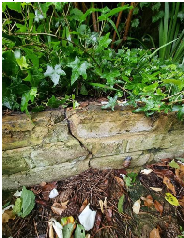
Photo 3. Displaced dwarf wall
