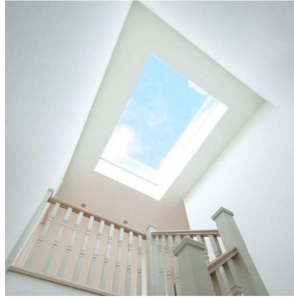
Flat roof skylight
