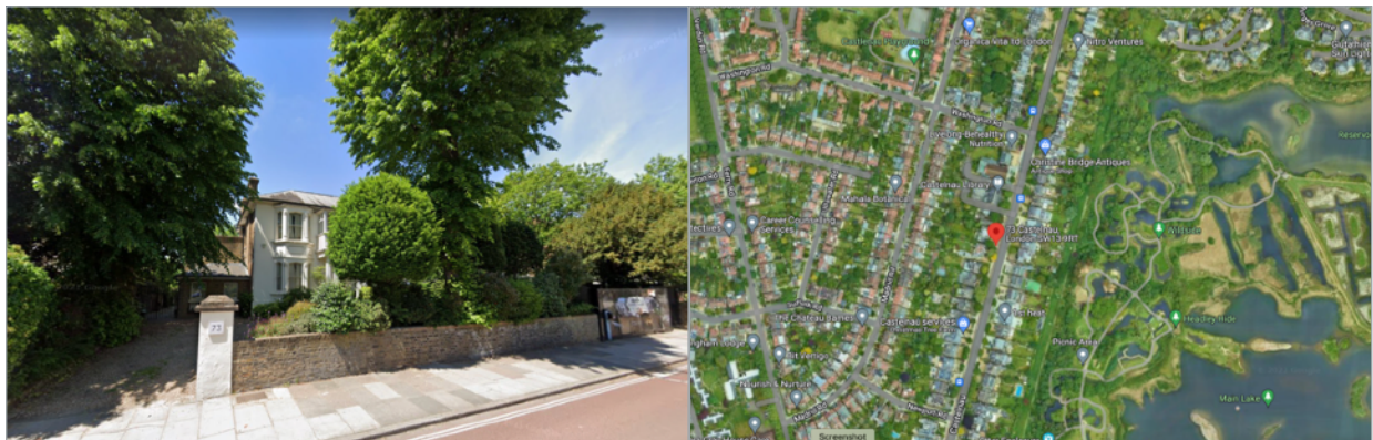
Street view (left) and aerial view (right) of 73 Castelnau. Source: Google Maps
