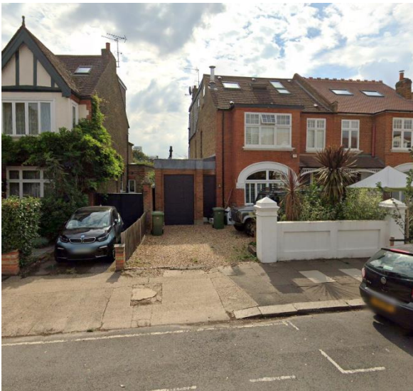
Figure 8 – Existing Frontage at 34 Nassau Road
