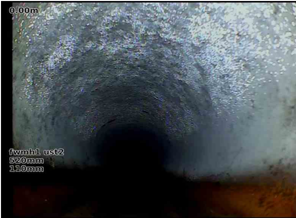
fwmh1 ust2X_127f8755-9e42-43df-b262-c778cd27fb33_20240207_230217_398.jpg, 00:00:00, 0.00 m Start node, manhole, reference: fwmh1 ust2
