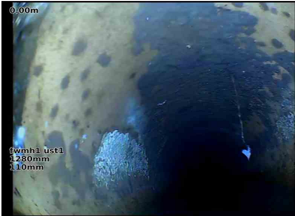
fwmh1 ust1X_050c8132-337f-40a8-9bdd-d4d7d3cf4e33_20240207_22 5913_935.jpg, 00:00:00, 0.00 m Start node, manhole, reference: fwmh1 ust1
