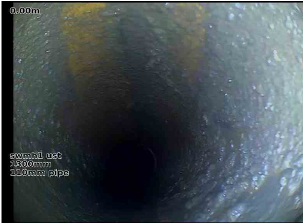
swmh1 ustX_575e0cbc-3c57-432e-9542-33f1bea78013_20240207_221 616_731.jpg, 00:00:00, 0.00 m Start node, manhole, reference: swmh1 ust
