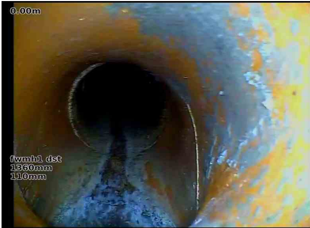
fwmh1 dstX_b4e23b4b-b114-4f0f-874c-64836493a88c_20240207_223 518_988.jpg, 00:00:00, 0.00 m Start node, manhole, reference: fwmh1 dst
