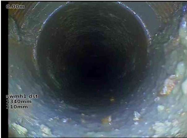
swmh1 dstX_6a475711-0d06-4ae5-8729-b93e5636e4bb_20240207_22 3101_845.jpg, 00:00:00, 0.00 m Start node, manhole, reference: swmh1 dst
