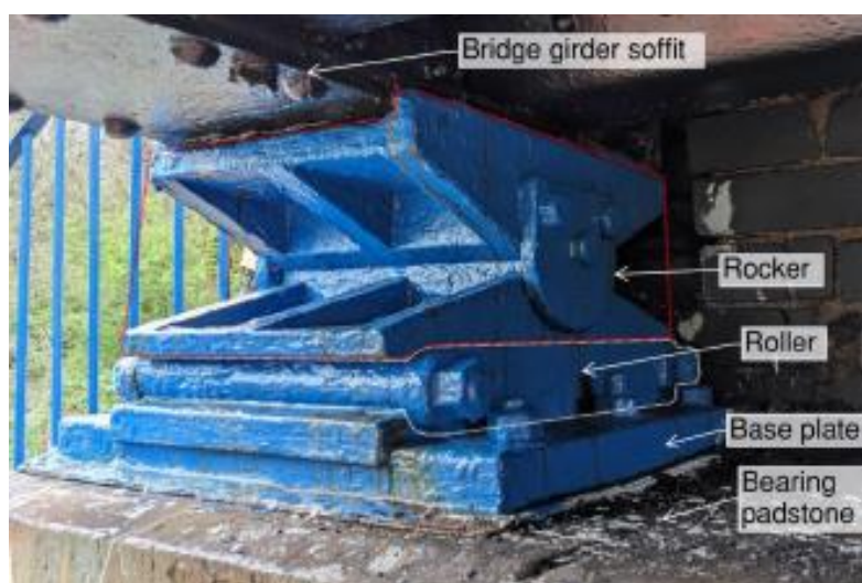
Figure 6 – Existing bearing arrangement
