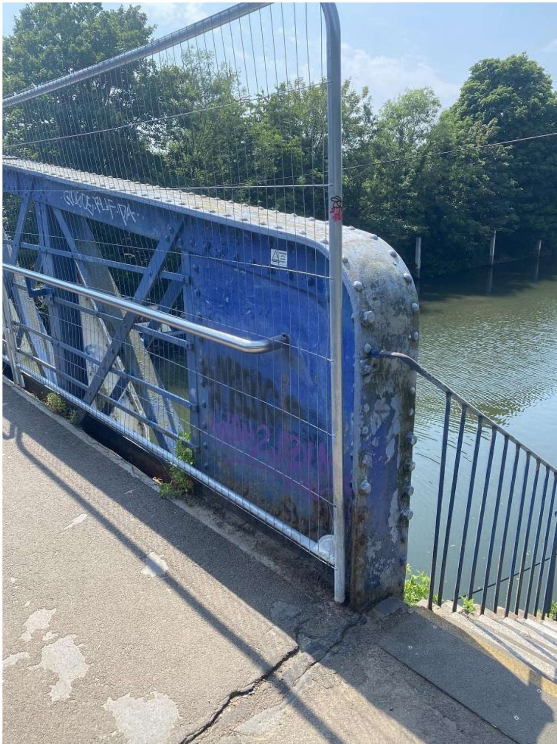
Plate 2. Lock Cut bridge, west parapet
