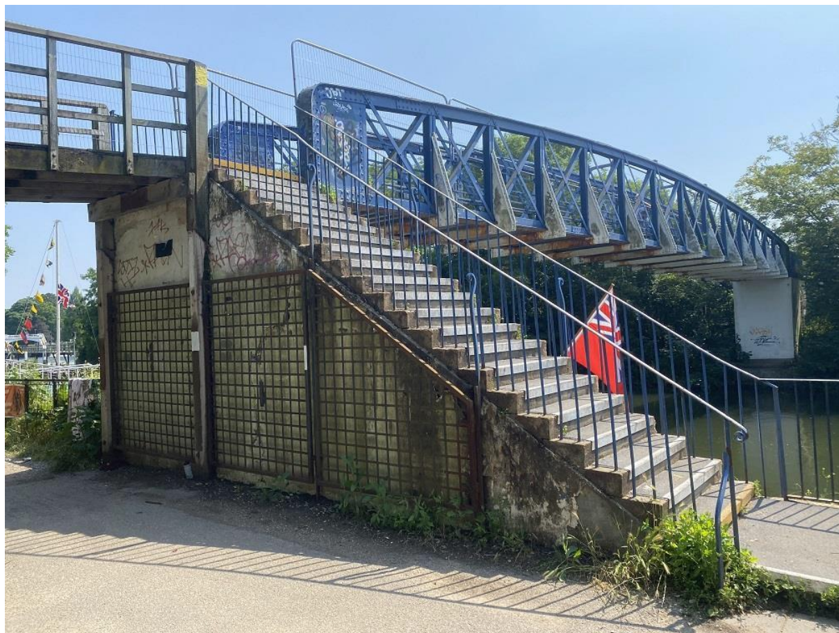
Plate 1. Lock Cut bridge, general view from Ham bank
