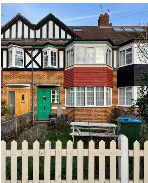
Figure 1 - Front View of 28 Broughton Avenue
