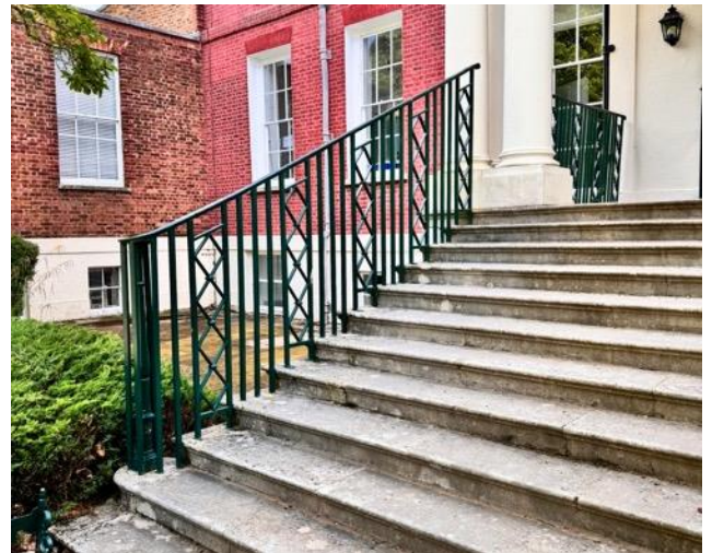
Existing railing style elsewhere in the building
