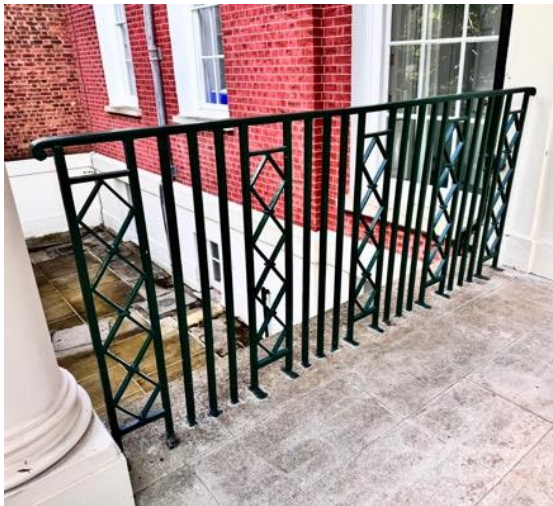
Existing railing style elsewhere in the building
