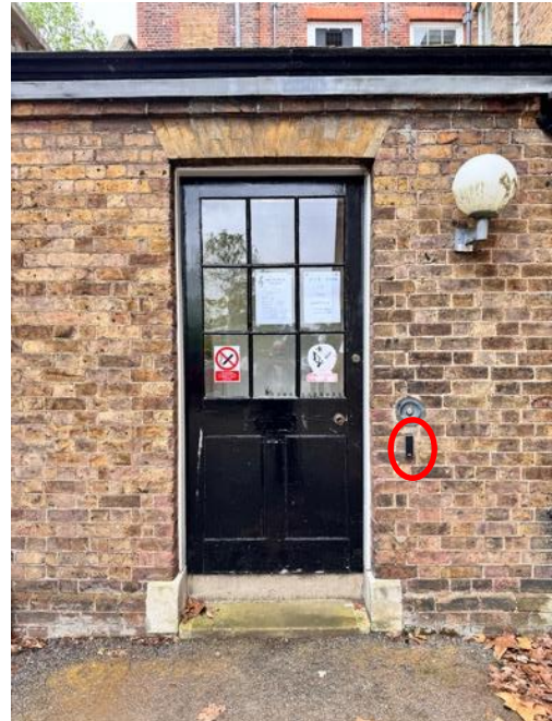
Existing Annex Door with access control externally
