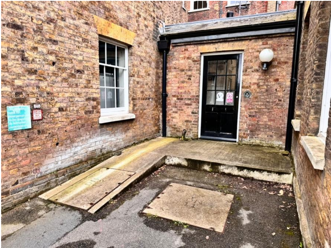
Existing ramp to be remodelled and new railings installed (railings to match existing style elsewhere in the building – see below).
