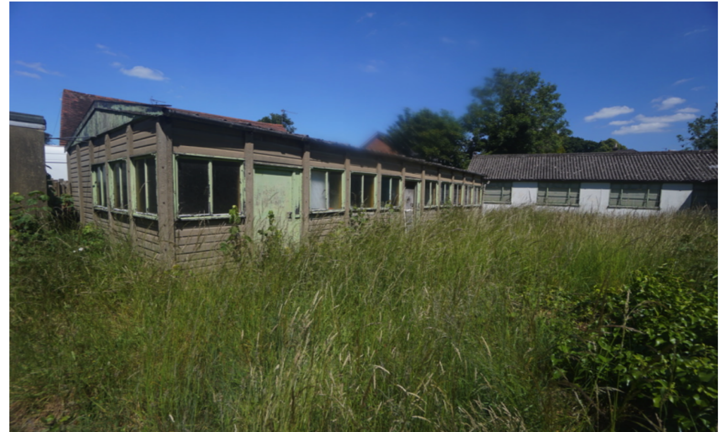
Figure 5: The Existing Site Photographs
