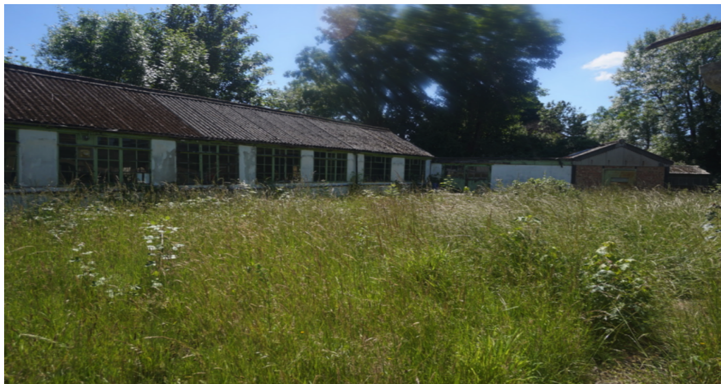
Figure 4: The Existing Site Photographs
