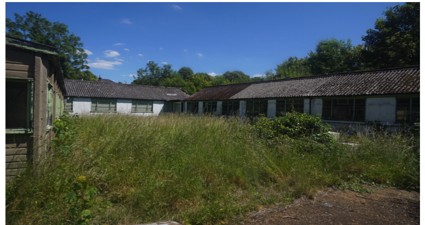
Figure 6: The Existing Site Photographs
