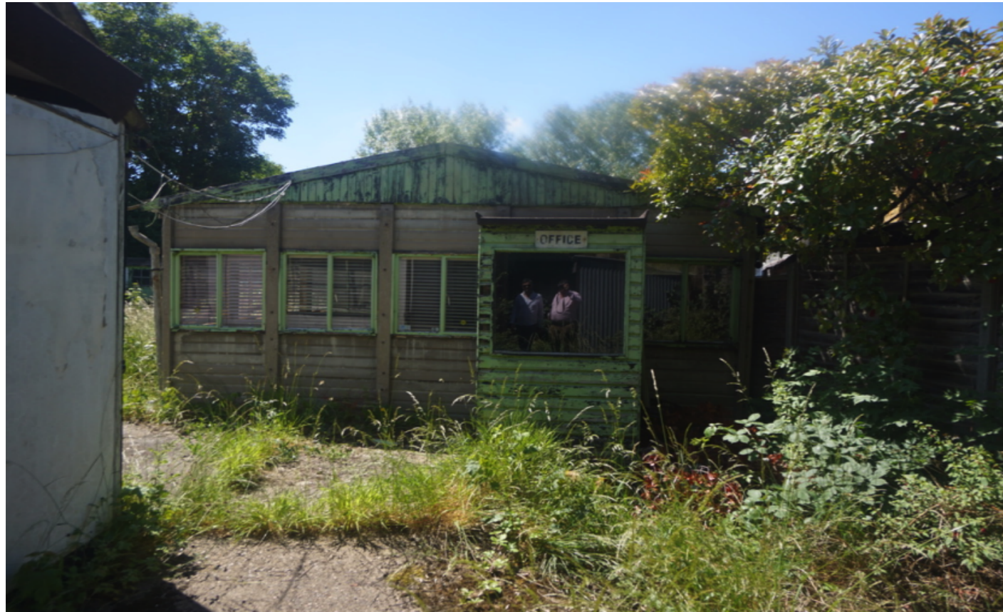
Figure 3: The Existing Site Photographs
