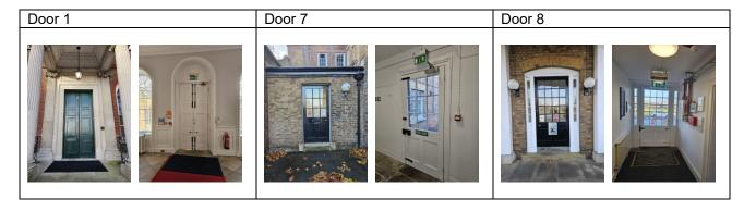
The exit mechanisms should be adjacent to the door but kept separate from the fire alarm call points and have it made perfectly clear which is which to avoid unwanted operation of the fire alarm, it may be best to locate the green emergency box on the opening side of the door. The design of the entry system on the exterior of the building does not impact on fire safety issues.
