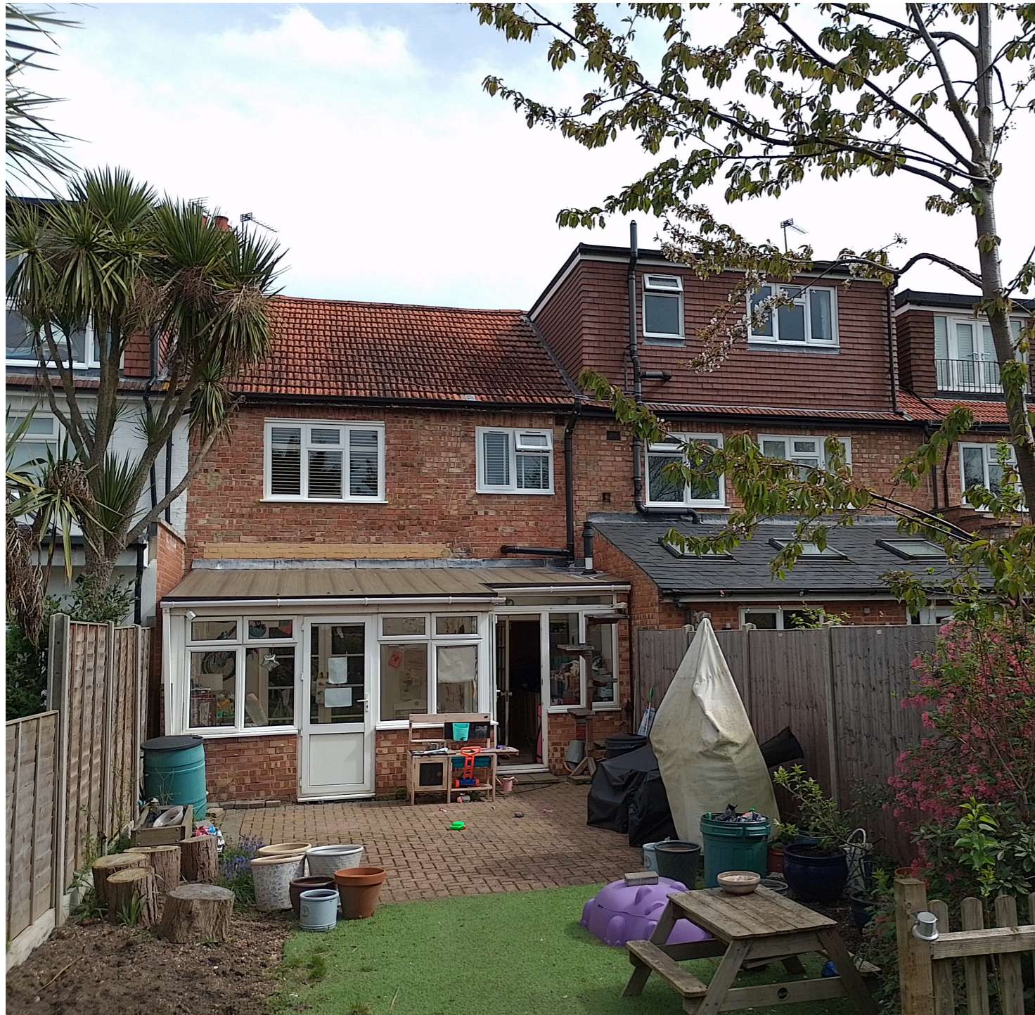
Site photograph: Existing rear elevation
