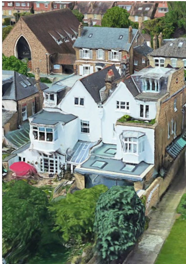
Figure 4: Aerial view of the rear Site (Google Earth) note extension at 80 Castelnau
