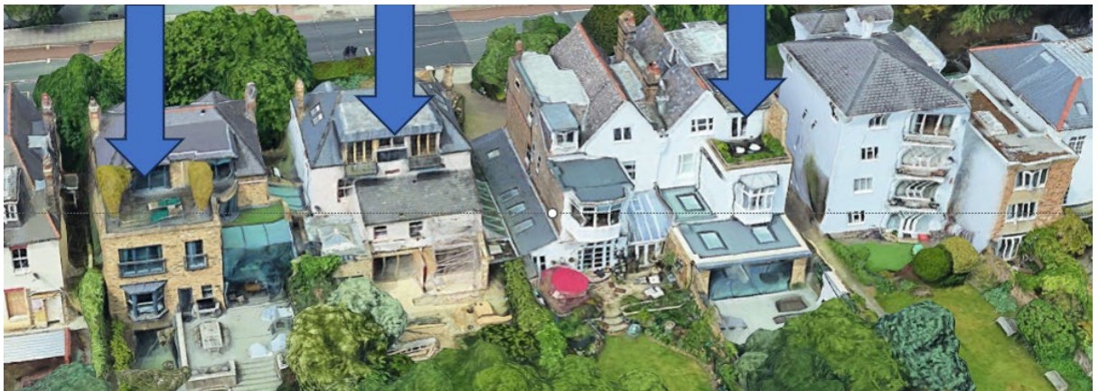
Figure 5: Aerial view of the rear of the Site (Google Earth) highlighting a number of properties with roof terraces
