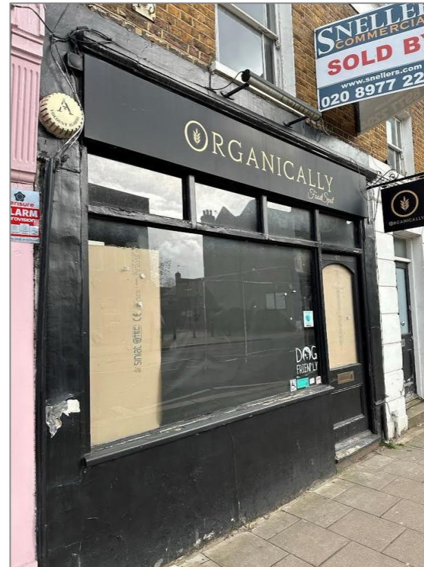
ORIGINAL FRONT ELEVATION SITE PICTURE
