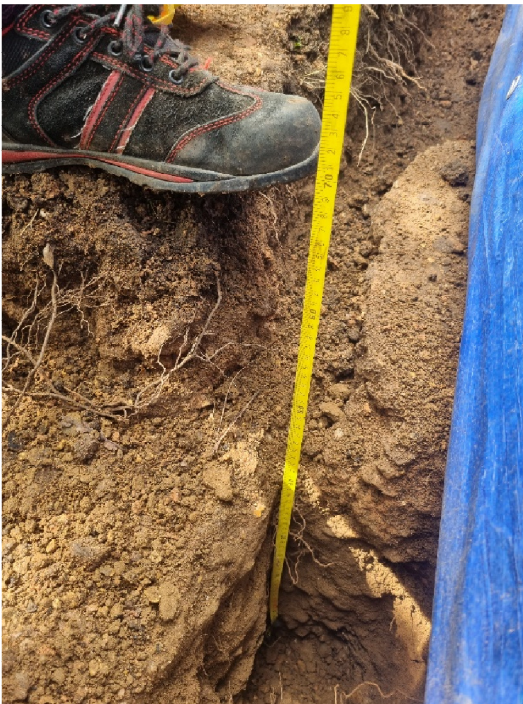
Figure 8: Depth of concrete recorded at 700mm.
