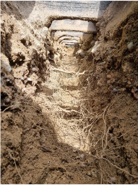
Figure 6: Extent of trench looking north. Fibrous roots from T45 present.
