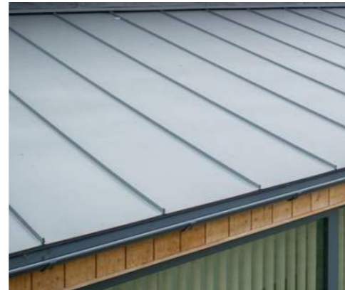
(Left) Pitched roof: Pre-weathered zinc standing seam roofing.
