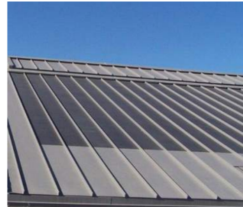
(Left) Pitched roof: Pre-weathered zinc standing seam roofing.
