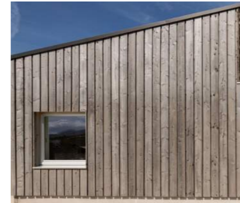
(Left) Upper parts of wall: Larch in a vertical board pattern, heat-treated or pre-coated to allow for even weathering.
