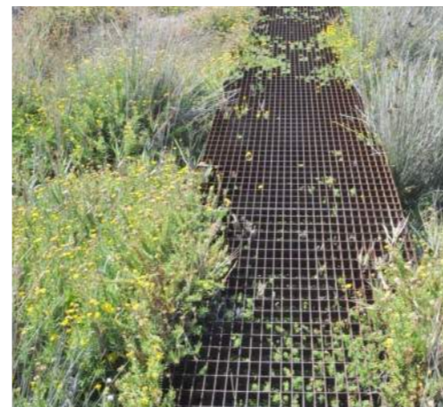
Mesh Bridge Across Swale
