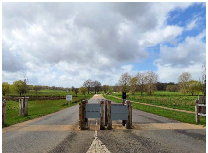
Main road view looking south-west from Roehampton Gate
