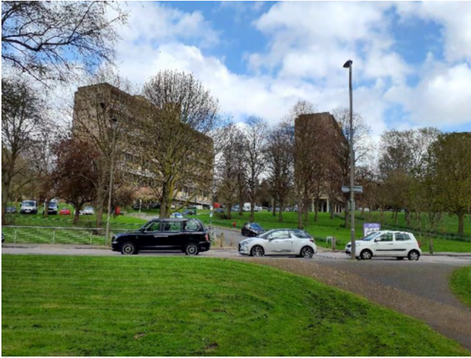
Photo taken from the south of the asset looking north
