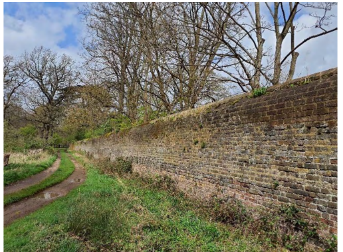
Figure 3.9 Boundary wall to the north of Roehampton Gate
