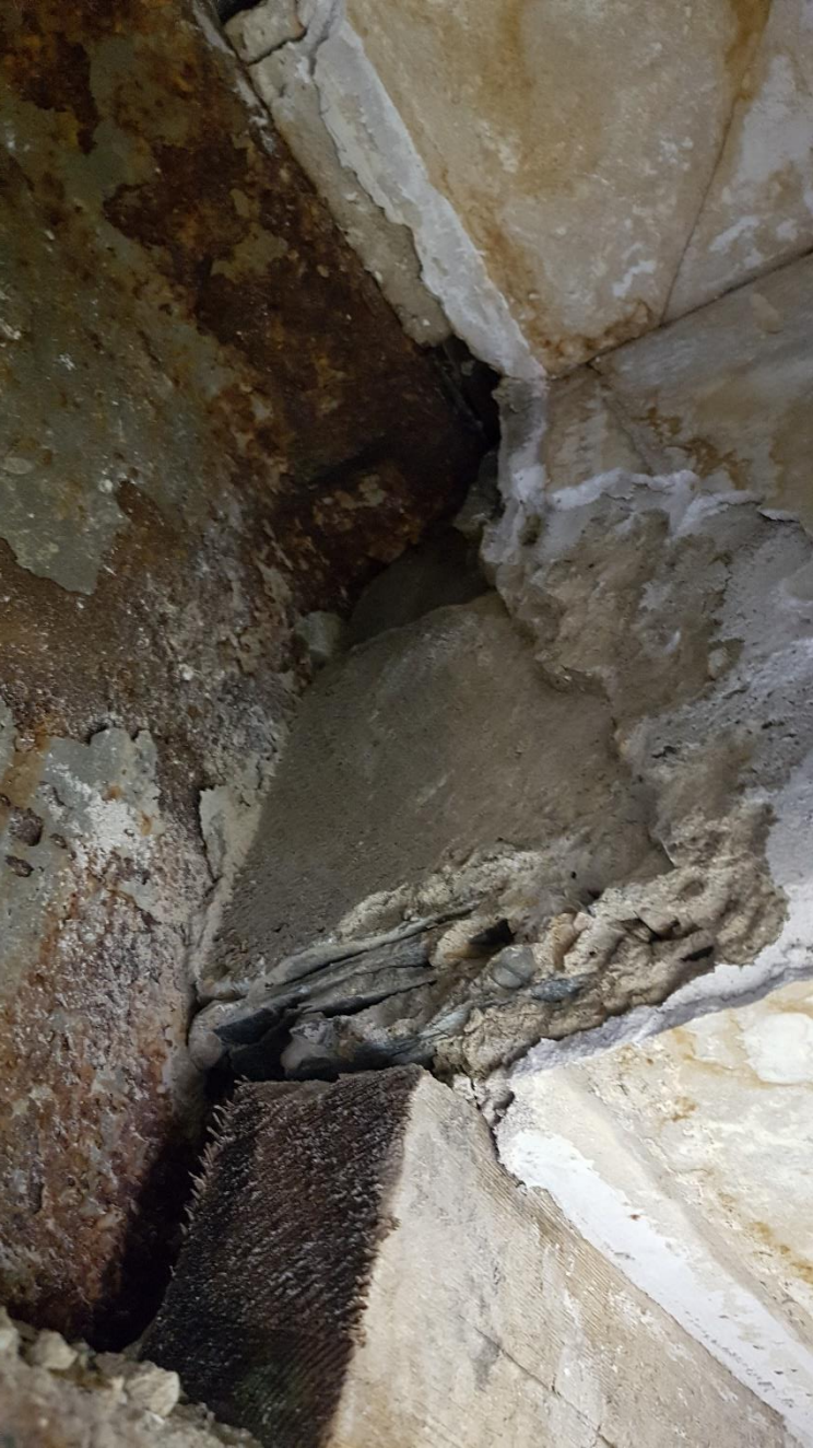
Photo 13 – Steel beams supporting concrete slab.
