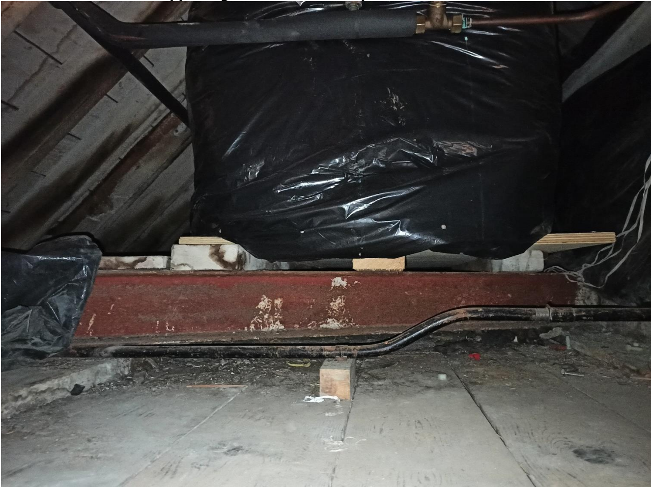
Photo 3 – Steel beams supporting water tank in loft space.
