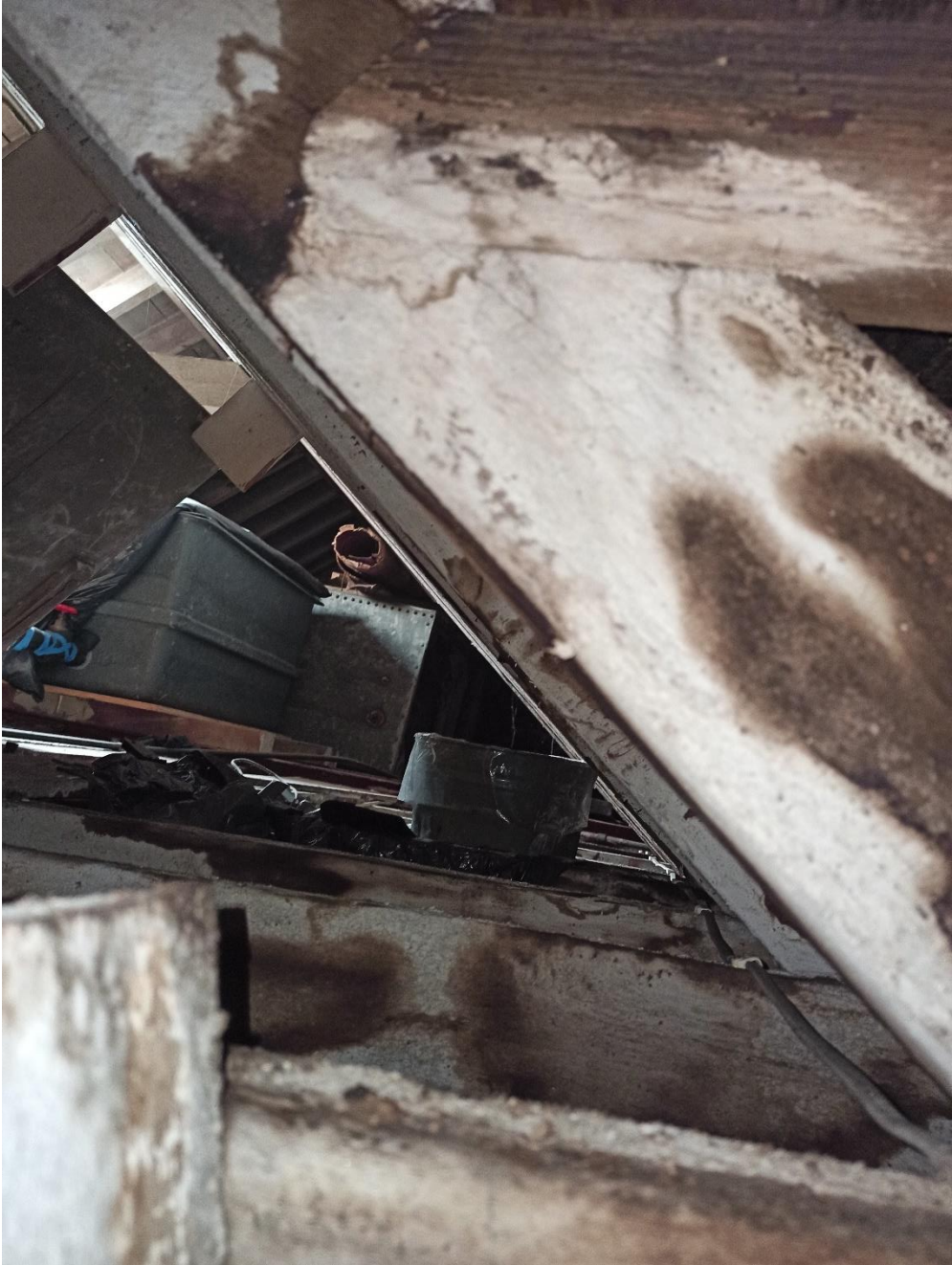
Photo 7 – Steel beams supporting water tank in loft space.
