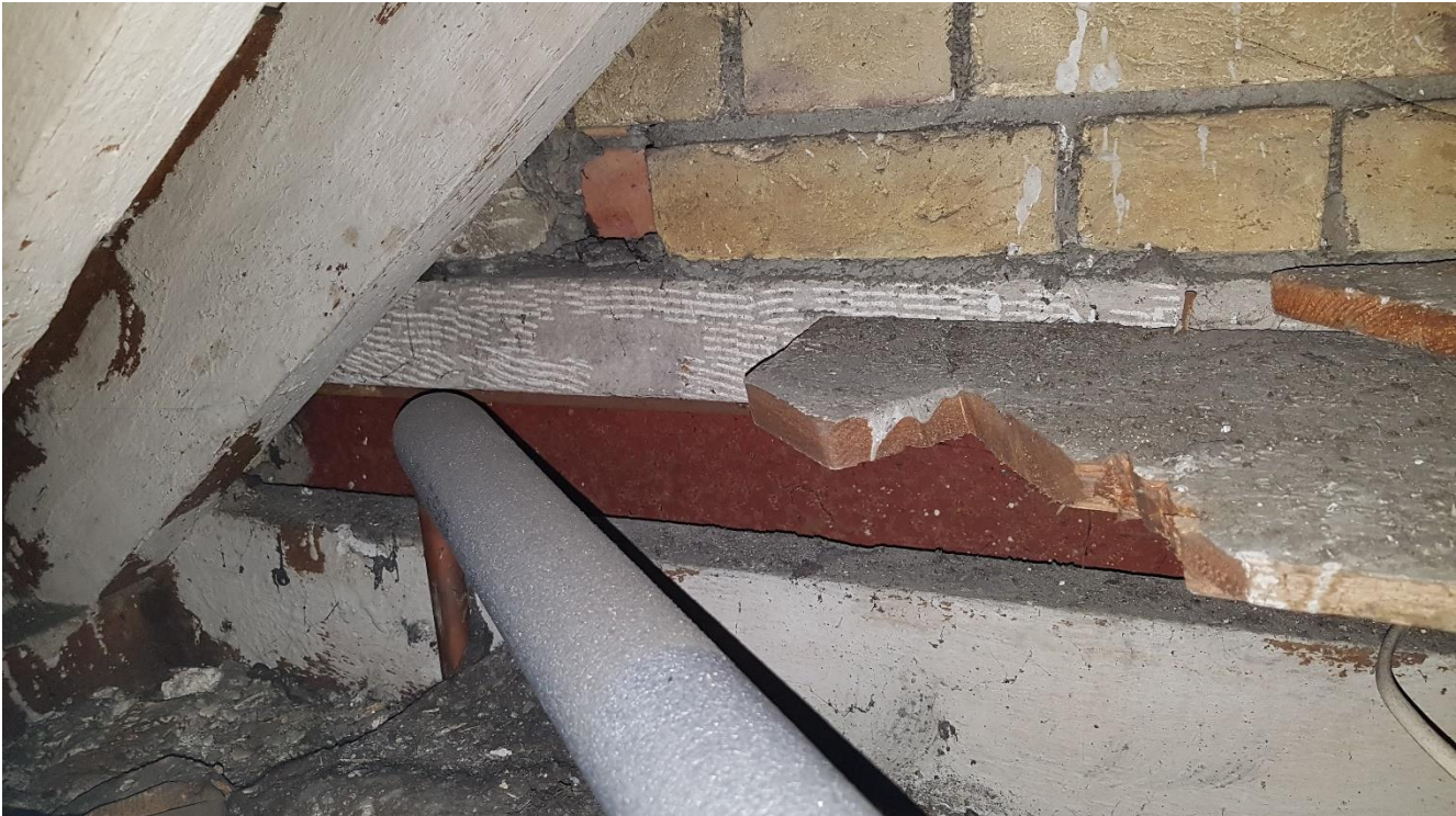
Photo 9 -Steel beam supporting above wall.
