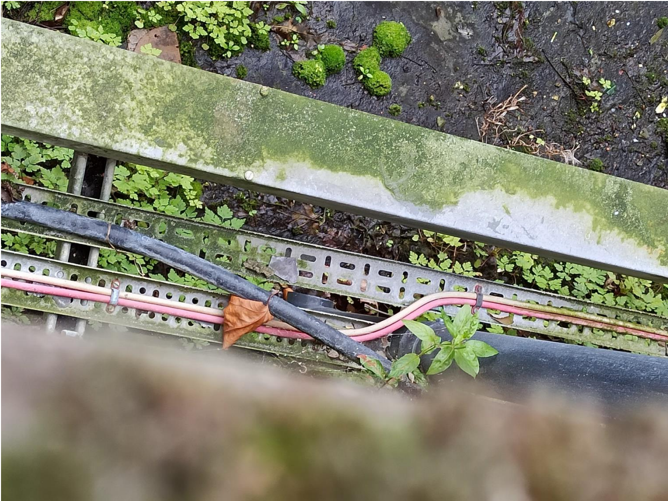
Photo 15 – Down pipe opening onto flat roof.
