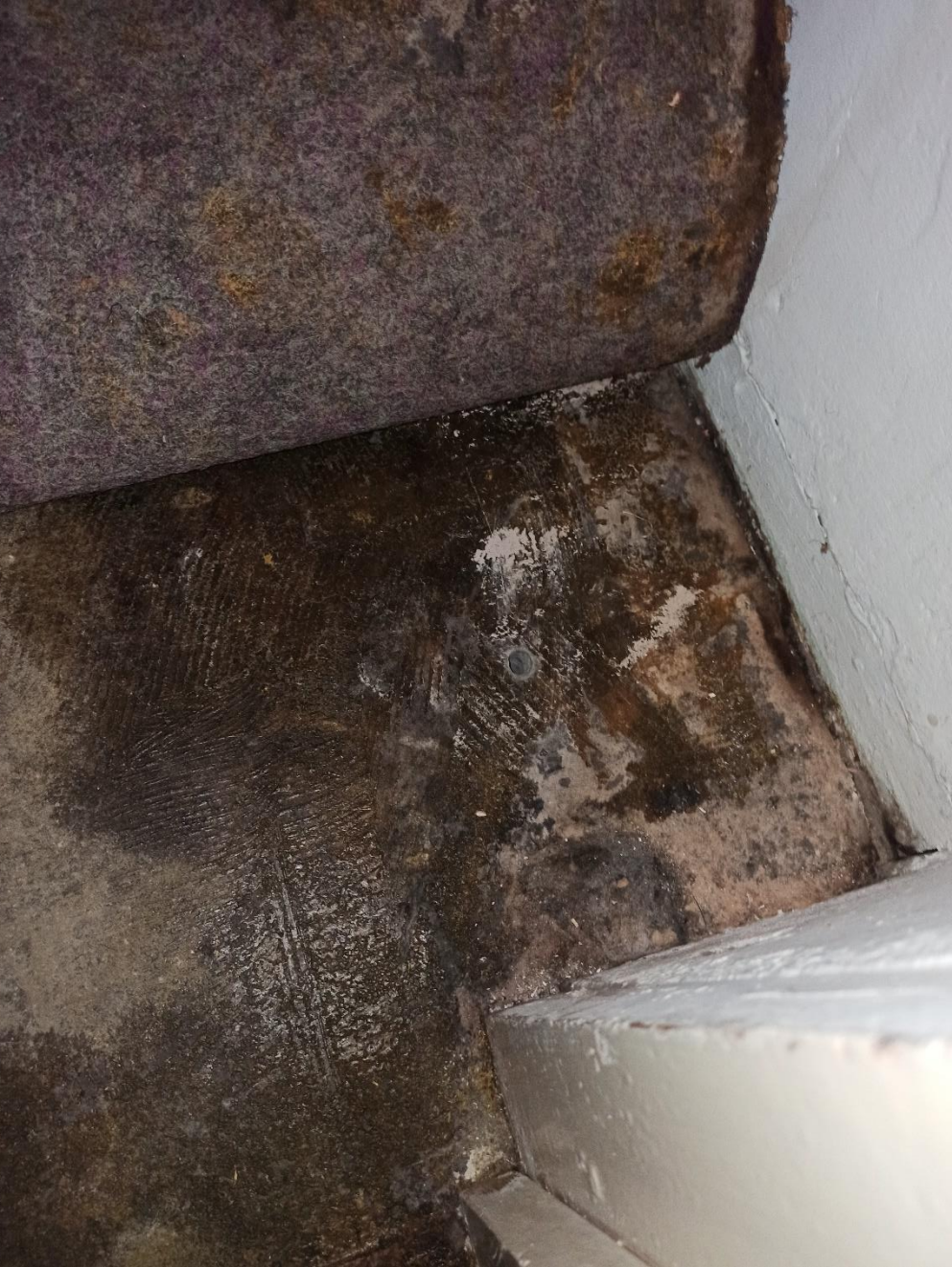
Photo 11 – Hole showing screed and concrete slab material.
