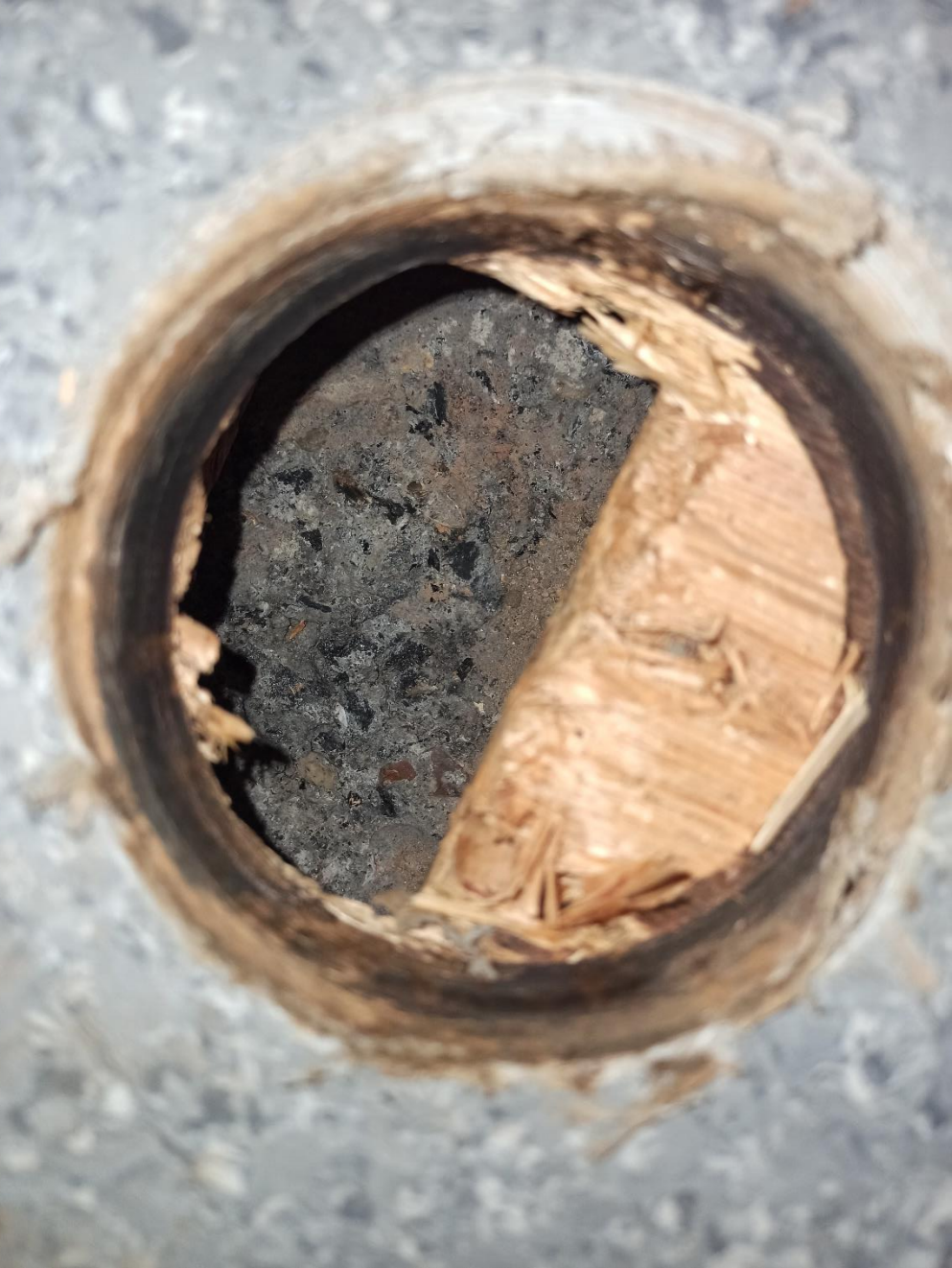
Photo 10 – Core showing floating timber floor over concrete slab.
