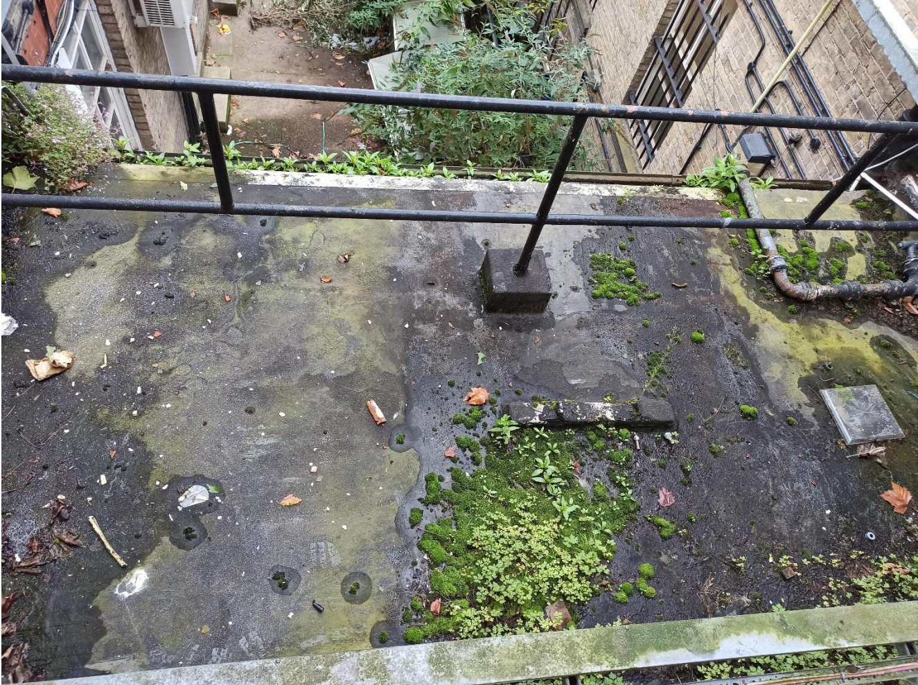
Photo 14 – Flat roof receiving rainwater from downpipes.
