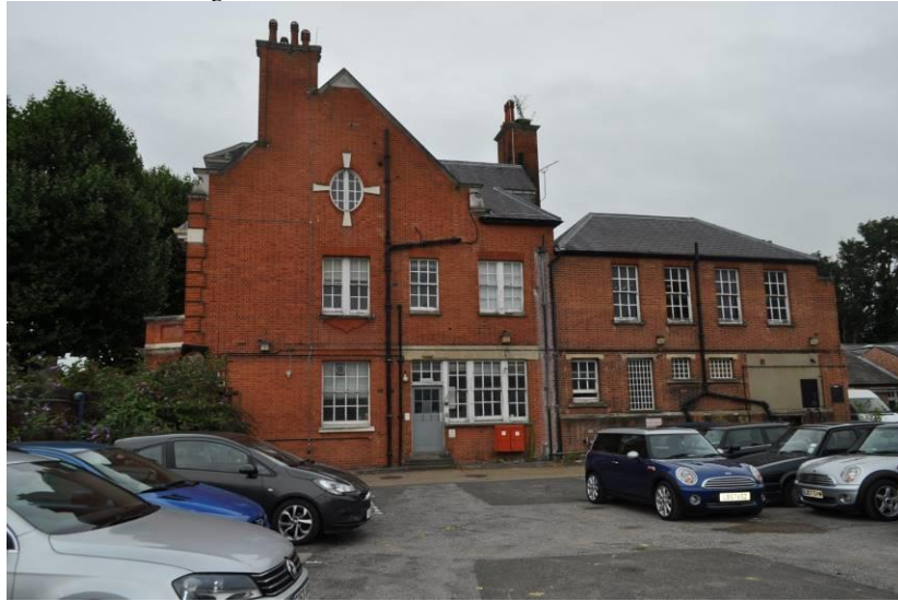
Plate B.1 Main Building - External
