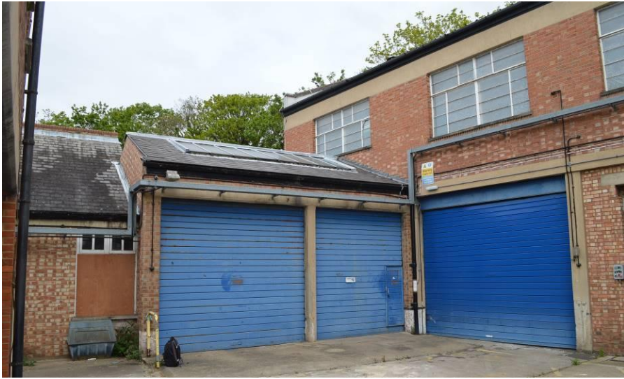
The 1930s sheds and garages in the north west corner of the site.
