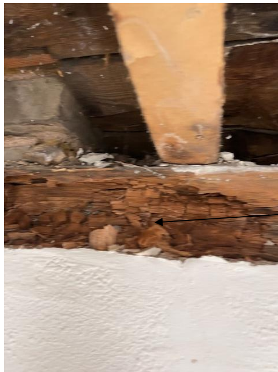
Photo 2 Close-up of decayed timbers
