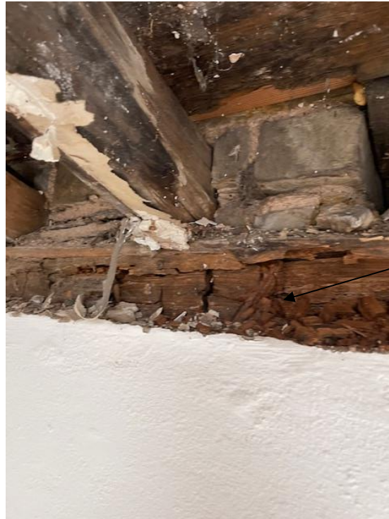
Photo 1 Rotted wallplate and rafter feet
