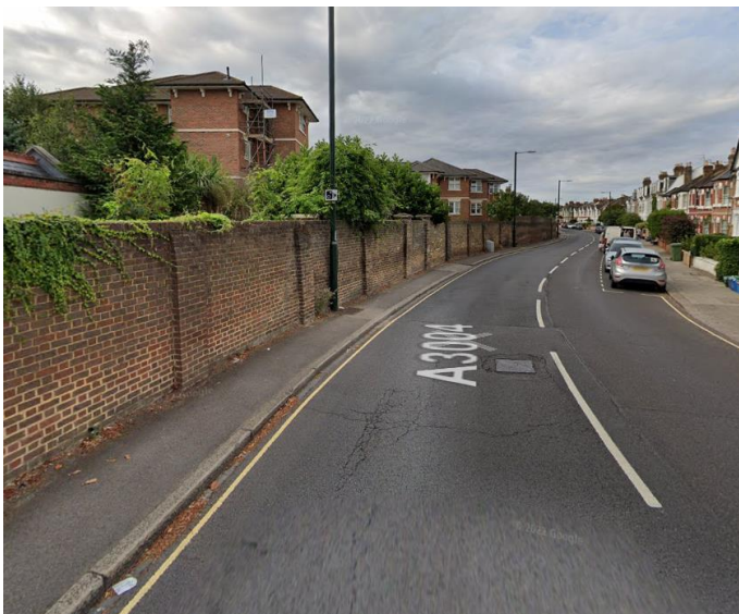
Image 3: Aerial image showing the site (source: Google Streetview)
