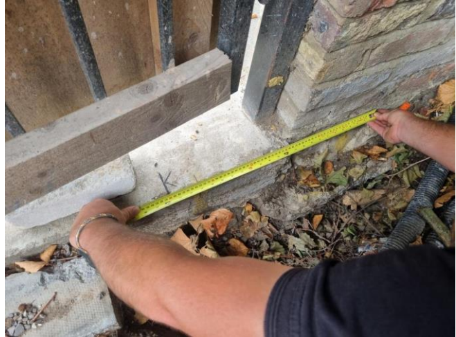
Photo 4. Position of TP2 along wall.
