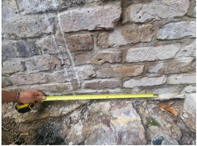
Photo 2. Position of TP1 along wall.
