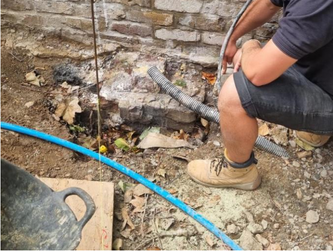
Photo 1. Location of TP1 (existing foundations exposed).
