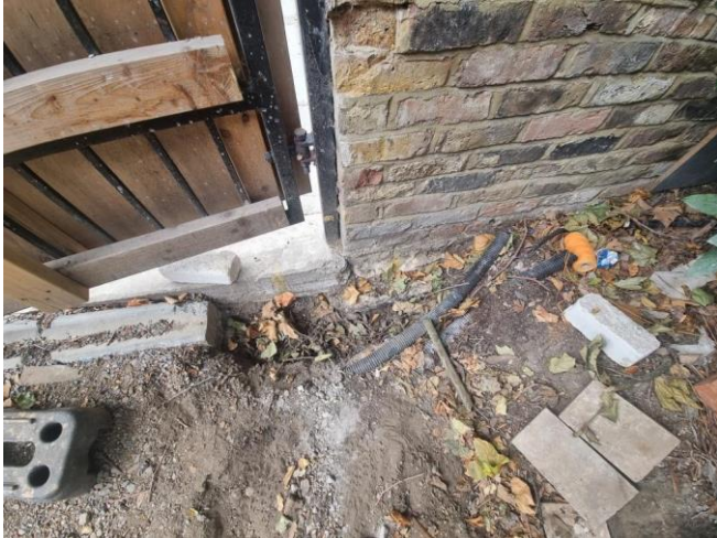
Photo 3. Location of TP2 (existing foundations exposed).
