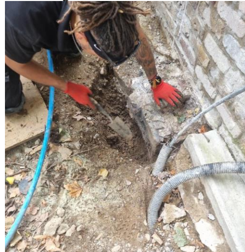
Photo 6. Using trowel to remove loose soil.
