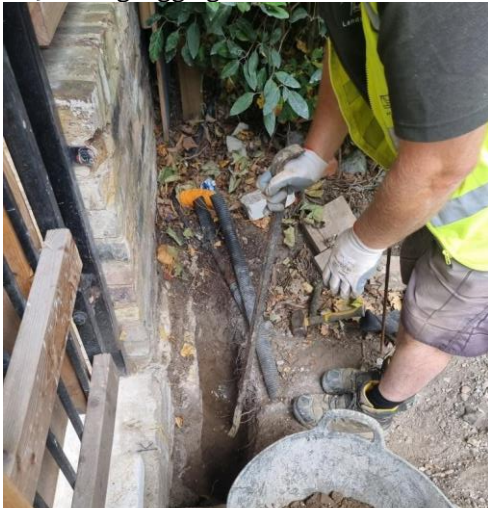
Photo 5. Using digging bar to loosen soil.
