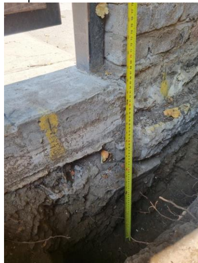
Photo 10. Tp2 after excavation.
