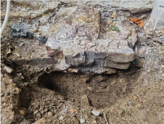
Photo 7. Tp1 after excavation.
