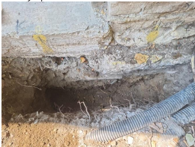
Photo 9. Tp2 after excavation.
