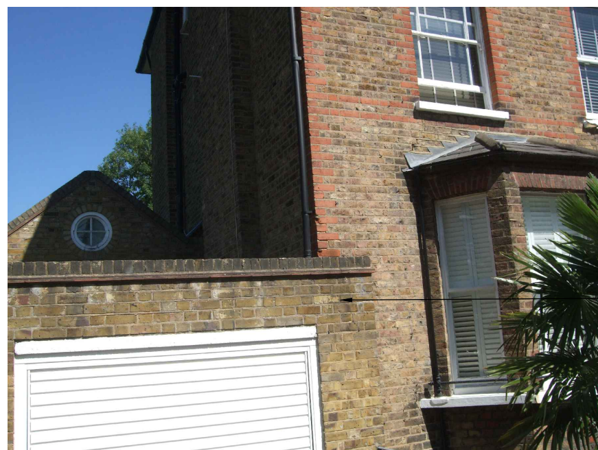
EXISTING GARAGE EXTENSION OF 50 THE VINEYARD PROTRUDES BEYOND MAIN BUILDING LINE - PROPOSED EXTENSION TO BE SET BACK BEHIND BUILDING LINE
